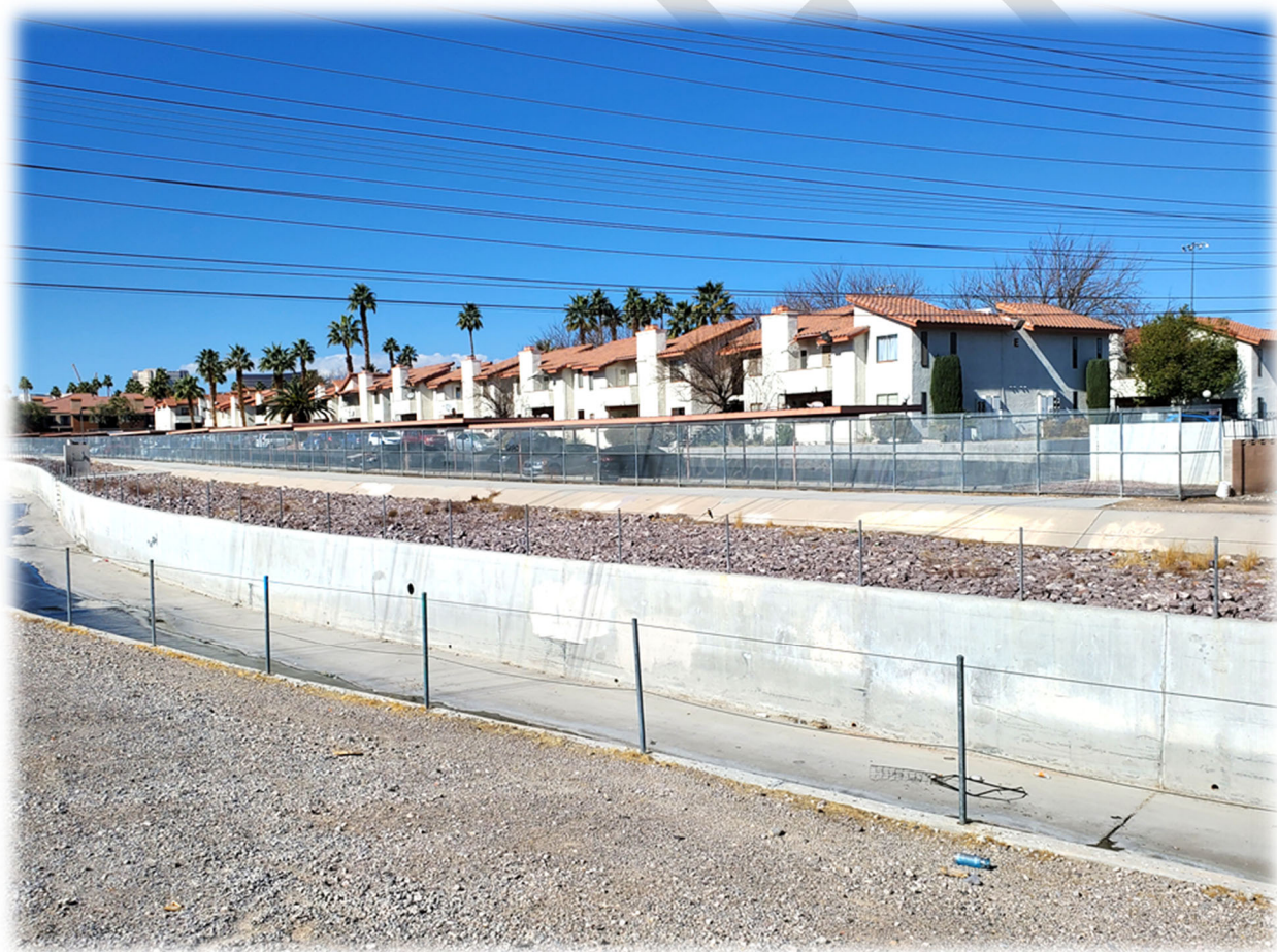
Figure 8. Flamingo Wash showing high fencing outside of maintenance road. Fencing and vertical concrete walls are meant to prevent people from entering into the channel.
