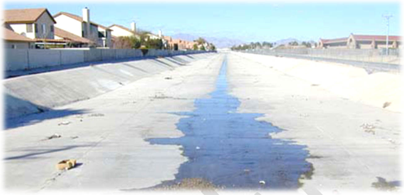
Figure 4. Engineered tributary channel in Las Vegas, showing dry-weather flow and a lack of habitat.
