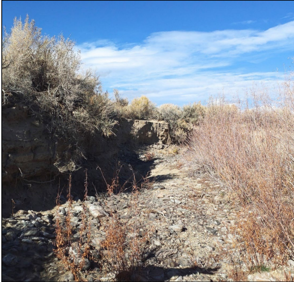
Figure 3-1. Channel instability/incision within the main stem of Peavine Creek.
