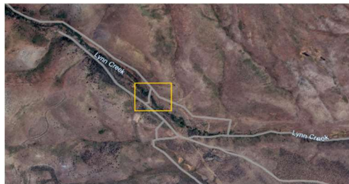
Fig 43. TU. The damaged culverts beneath vegetation cover on Lynn Creek. While not visible, four culverts are collapsed here. (June 2025).
