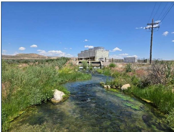
Fig 10. TU. The NGM water discharge site, including cooling
