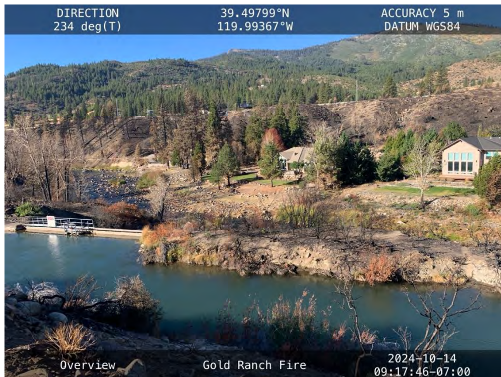
Photo 2: View of Priority Zone 1, showing steep slopes along the west side of the Truckee River. Photo taken on east side of TMWA Diversion with the view looking west. The burn area continues south along the west side of the Truckee River (not pictured).
