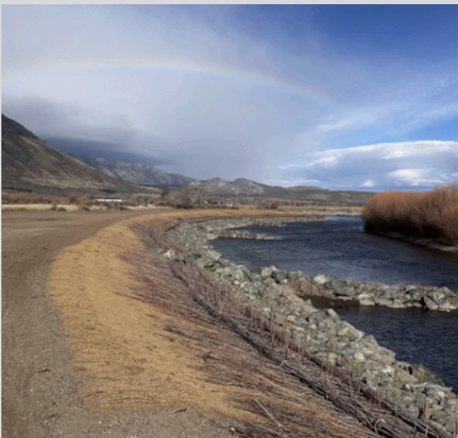
Streambank Stabilization Near Genoa
