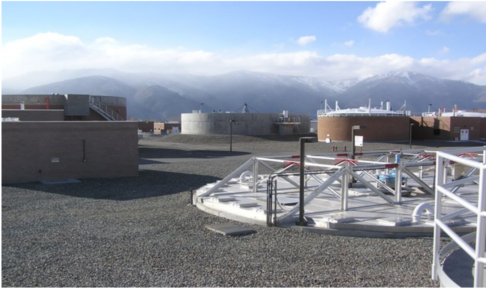
Minden Gardnerville Sanitation District wastewater energy co-generation enhancement
