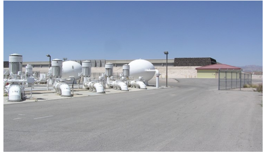
Las Vegas finished water reservoir rehabilitation
