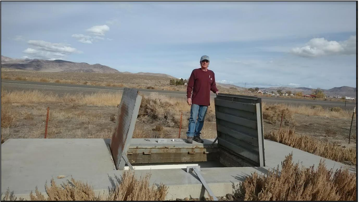
Staff showing the padlocked Vaults to distribution system adjacent to the highway
