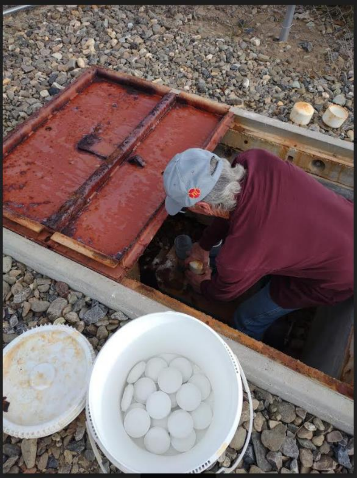
Current practice - Staff replacing the Chlorine tablet in the tubes placed over the water streaming from the stream (2021)
