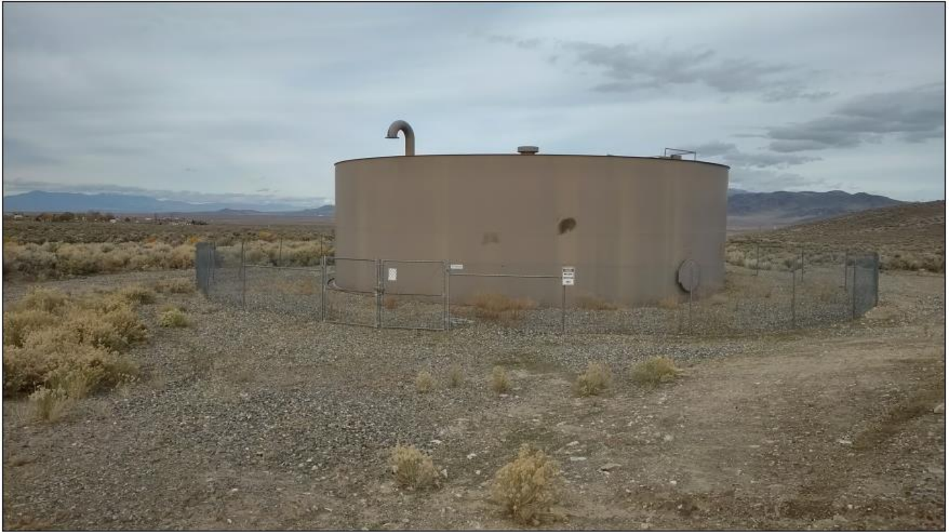
Storage Tank and Spring Overflow to the creek (2021)
