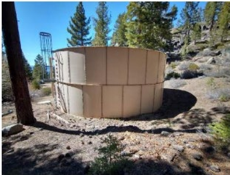
Existing Water Storage Tank (132,000 gallons, built 1969)
