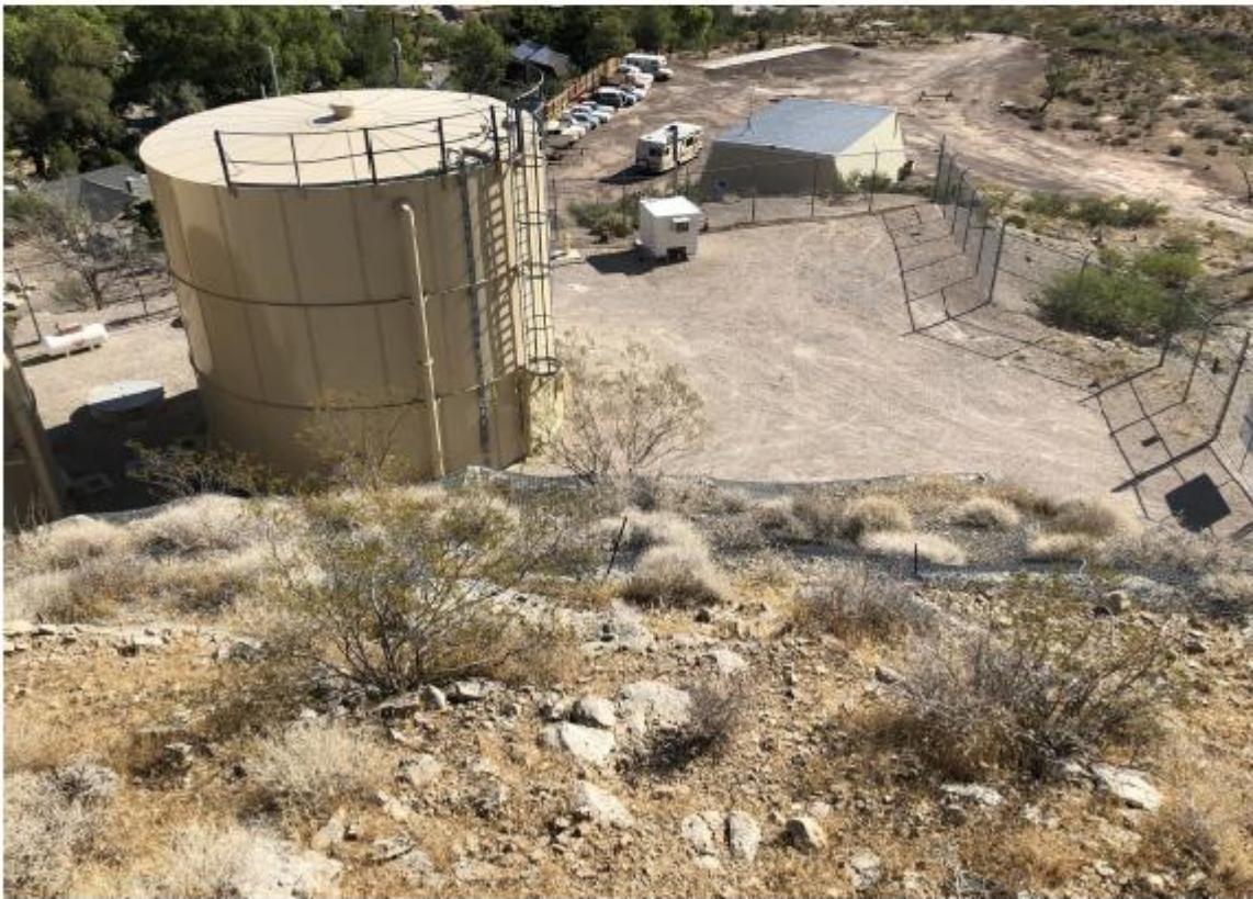
Site 5. Existing tank and partial view of proposed new tank site
