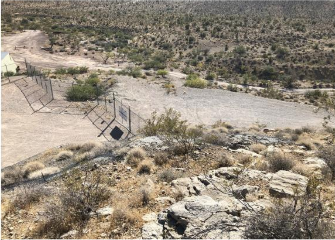
Site 5. New tank site
