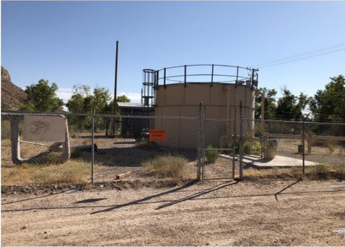
Site 1. Facing East at well site
