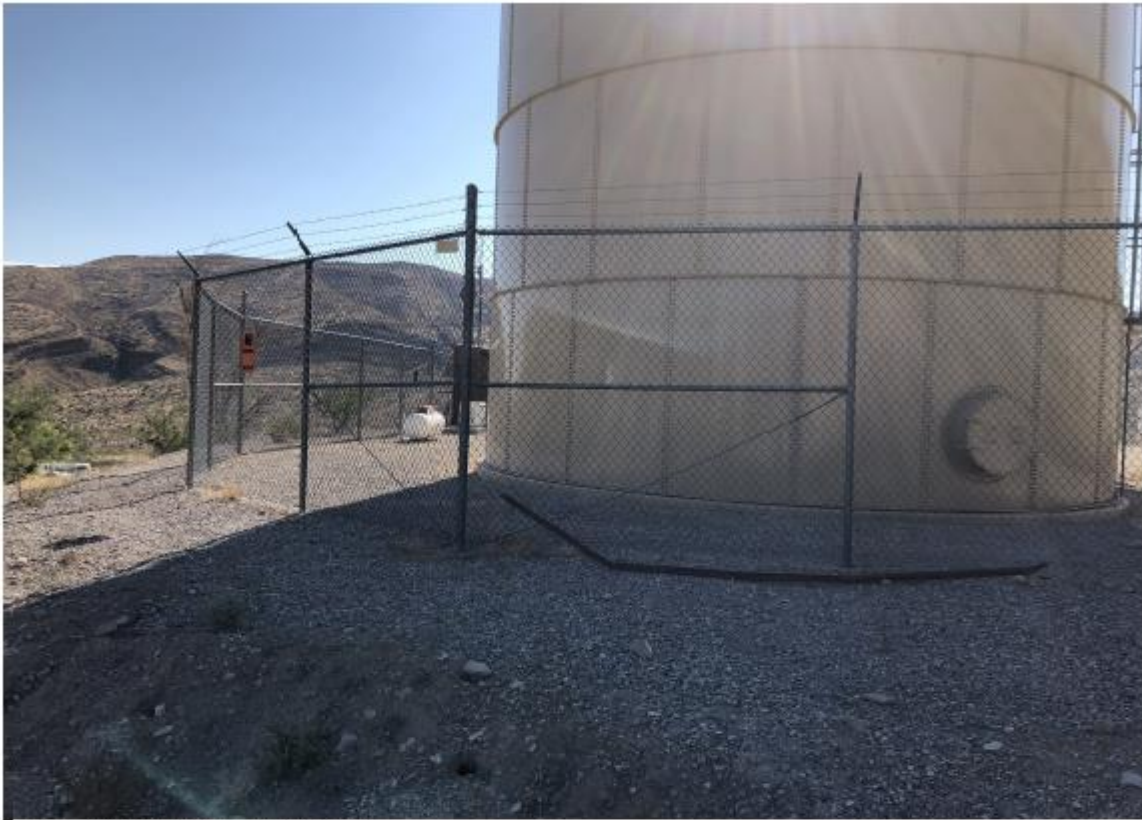
Site 5. Closeup of existing tank
