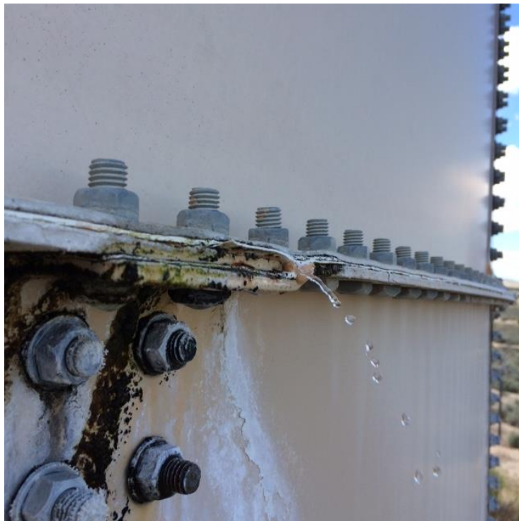
Old, leaking bolted-steel water tank
