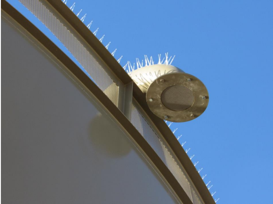
New, welded-steel, storage tank with BLM required perch deterrents & view screening
