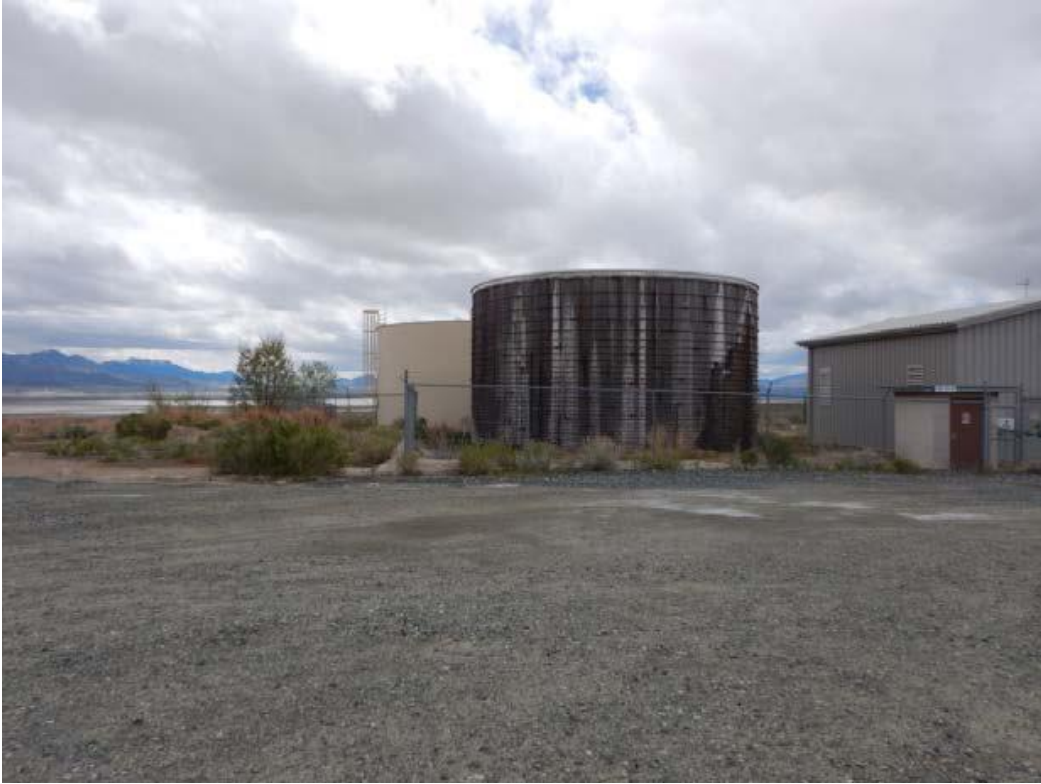
Raw water (redwood) and finished water (welded steel) tanks on uranium treatment site (Photo by Victor Villagran, SWCA)
