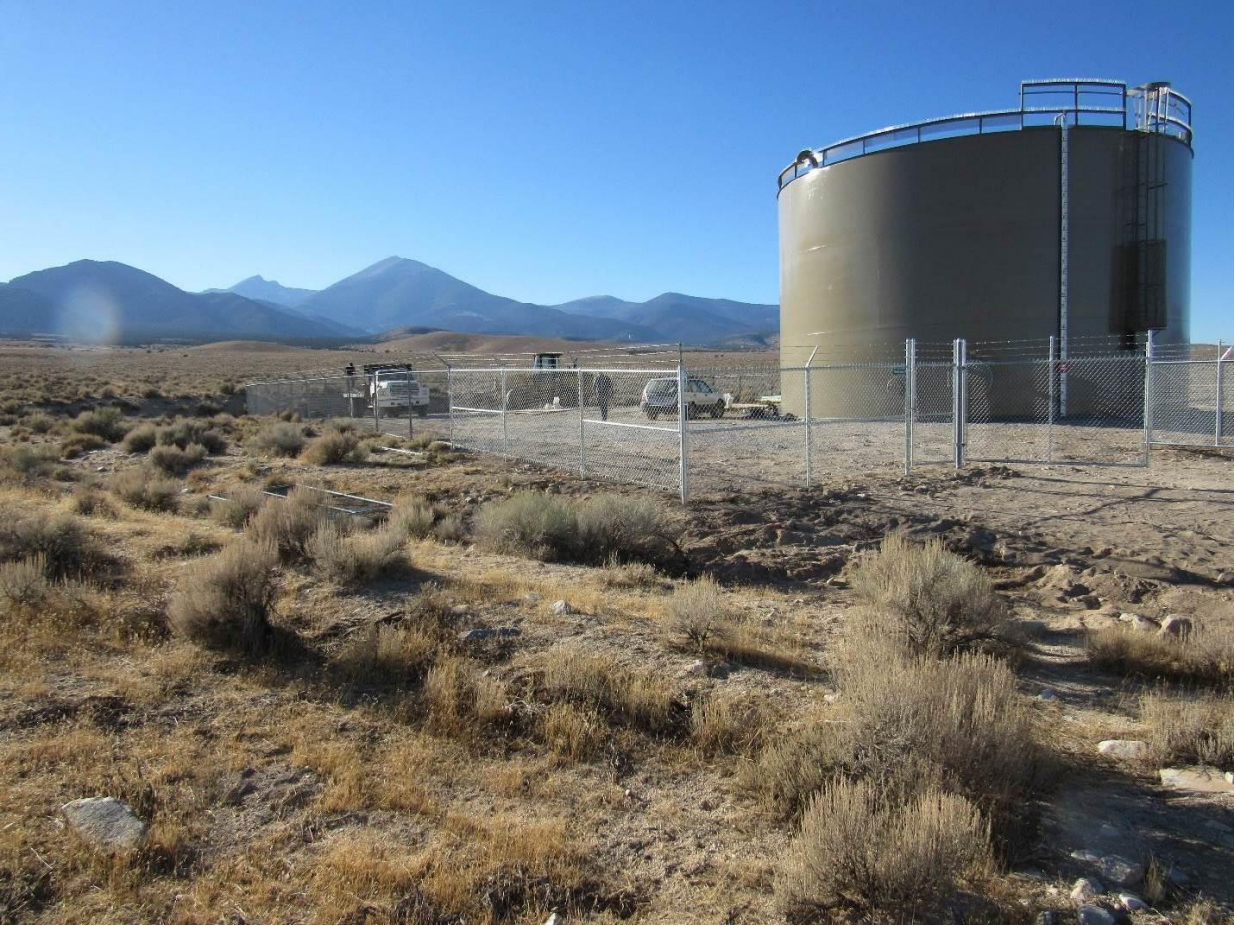
New, welded-steel, storage tank with BLM required perch deterrents & view screening
