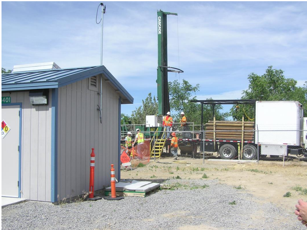
Sonic exploratory drilling
