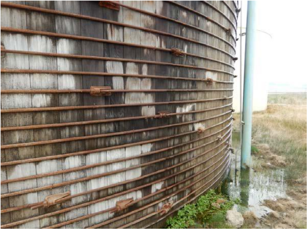
Water pooled at base of redwood tank (Photo by Victor Villagran, SWCA)
