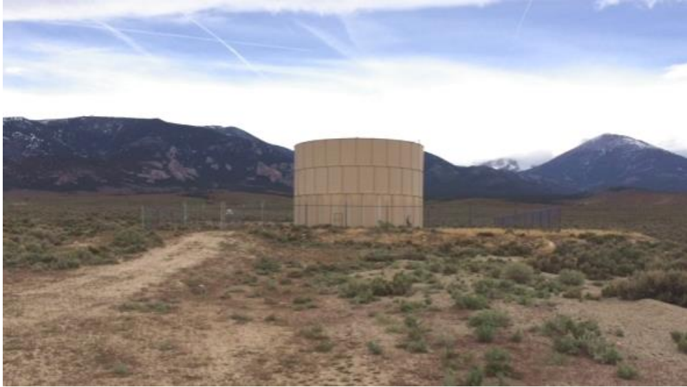
Old, leaking bolted-steel water tank
