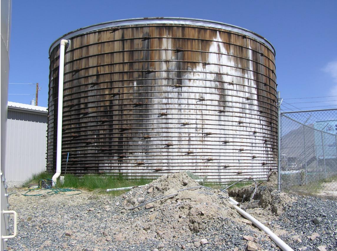
Raw water (redwood) tank
