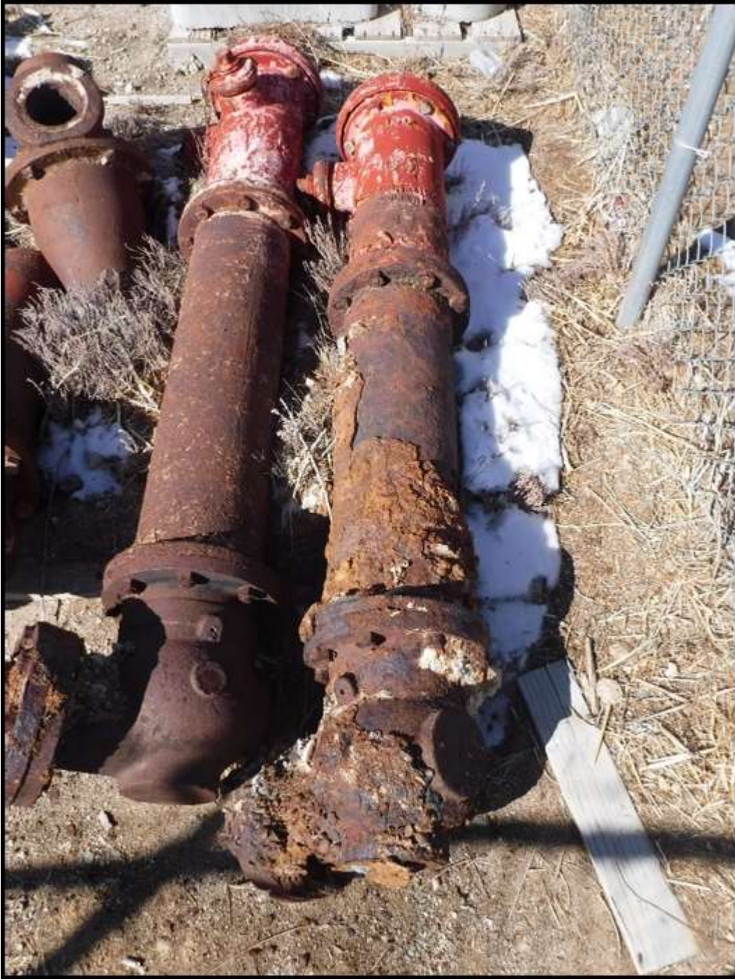
Corroded Shoe on Fire Hydrant (courtesy of Shaw Engineering)
