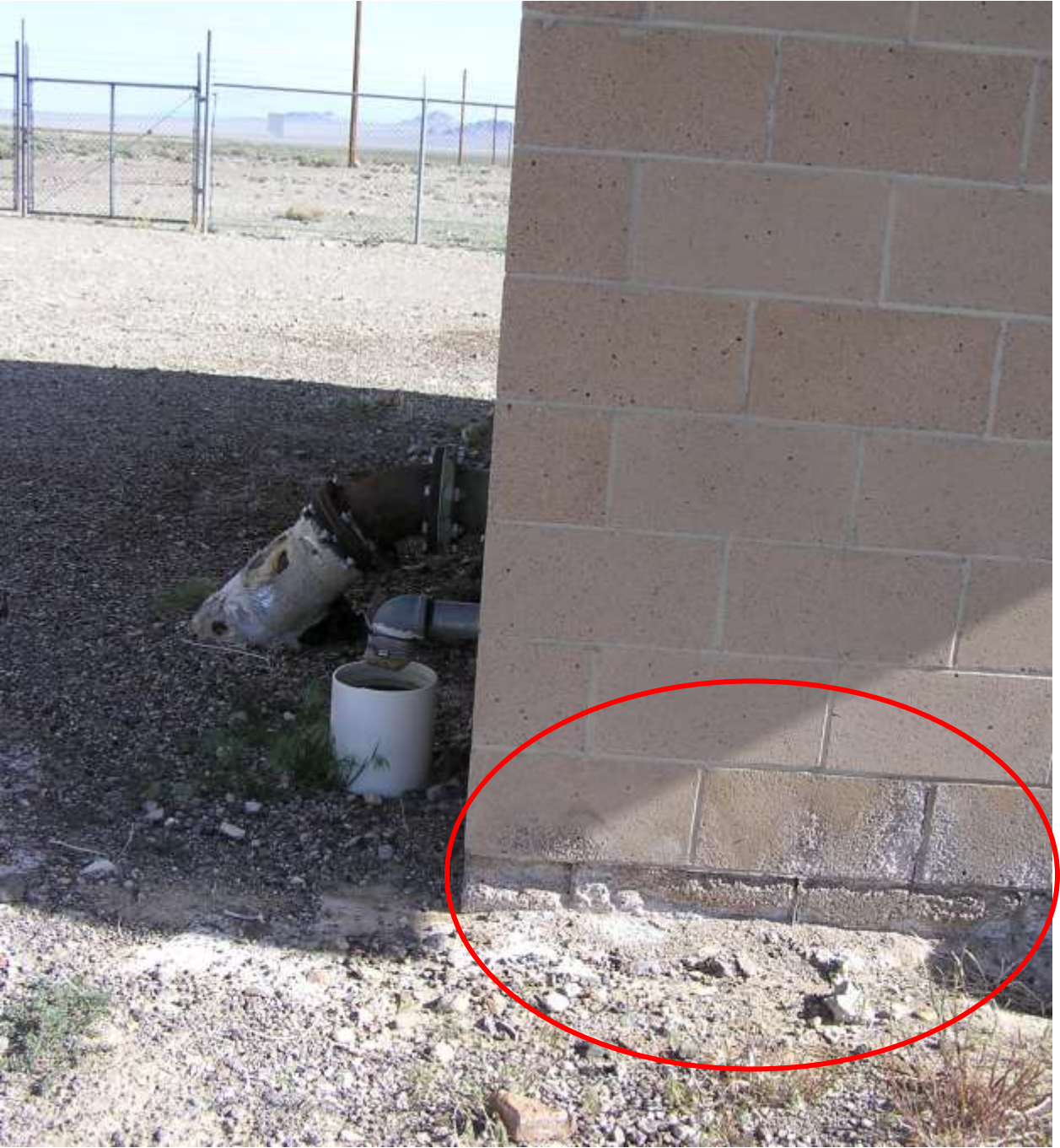
BPS 2 – Pump building erosion
