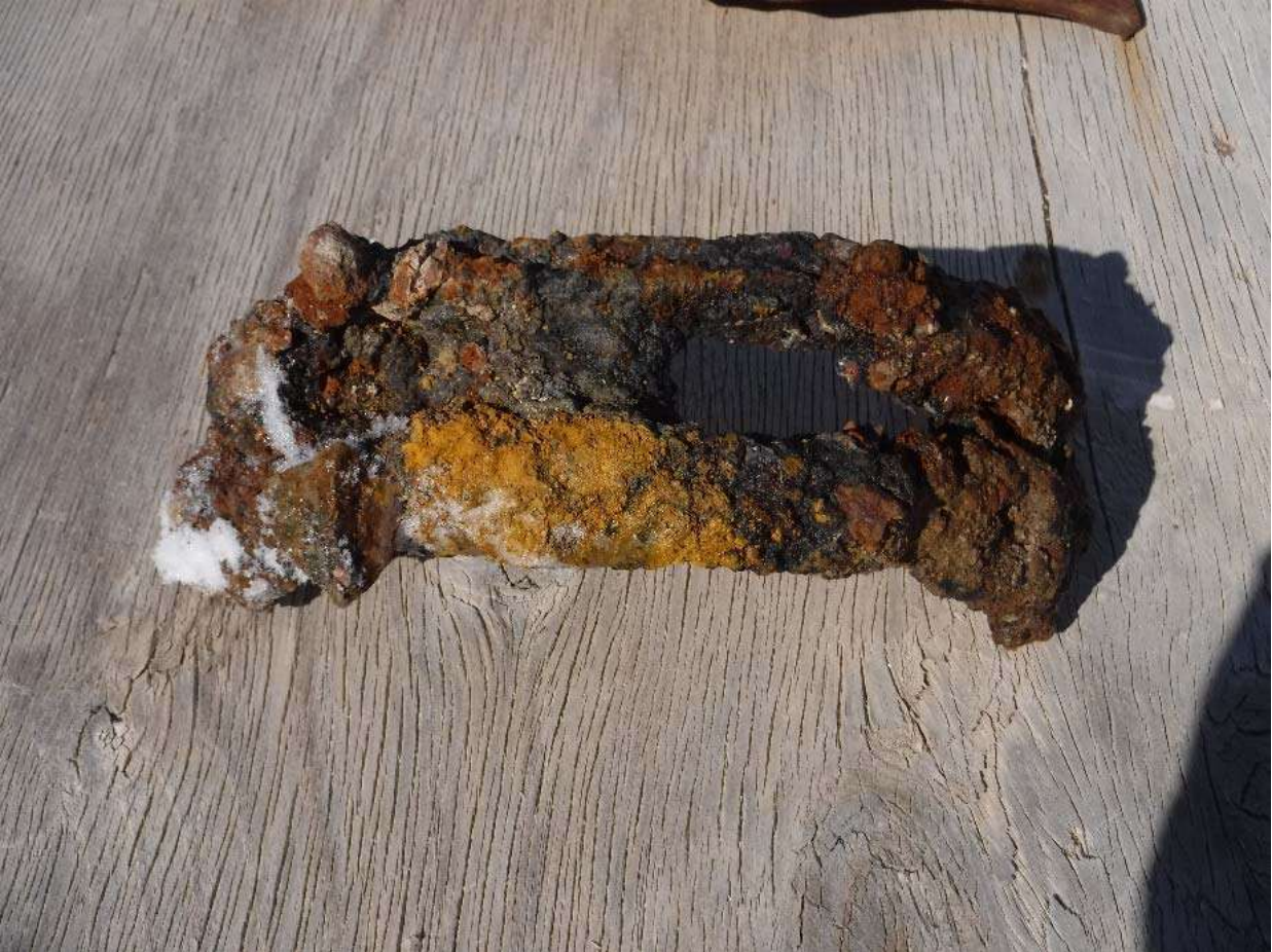
Corroded Water Service Saddle (courtesy of Shaw Engineering)
