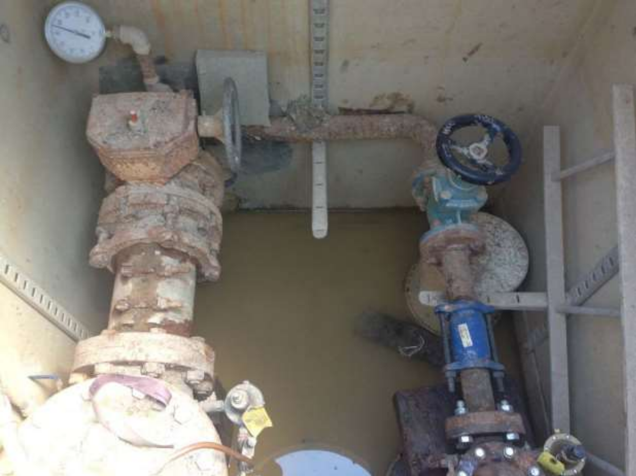
Existing Lower PRV Station. Note Pipe Corrosion and Standing Water (courtesy of Shaw Engineering)
