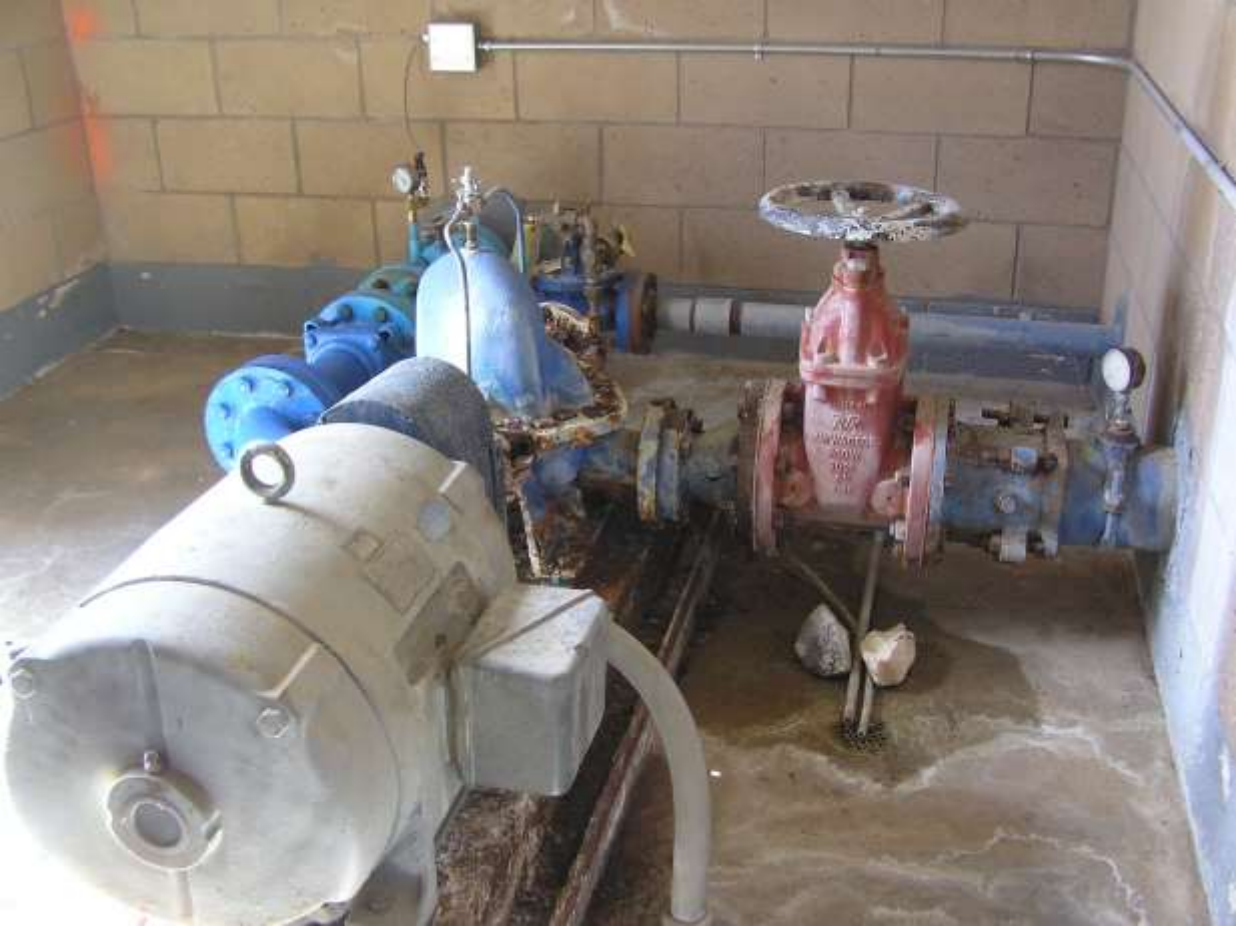
BPS 2 – Corrosion of pump & appurtenances
