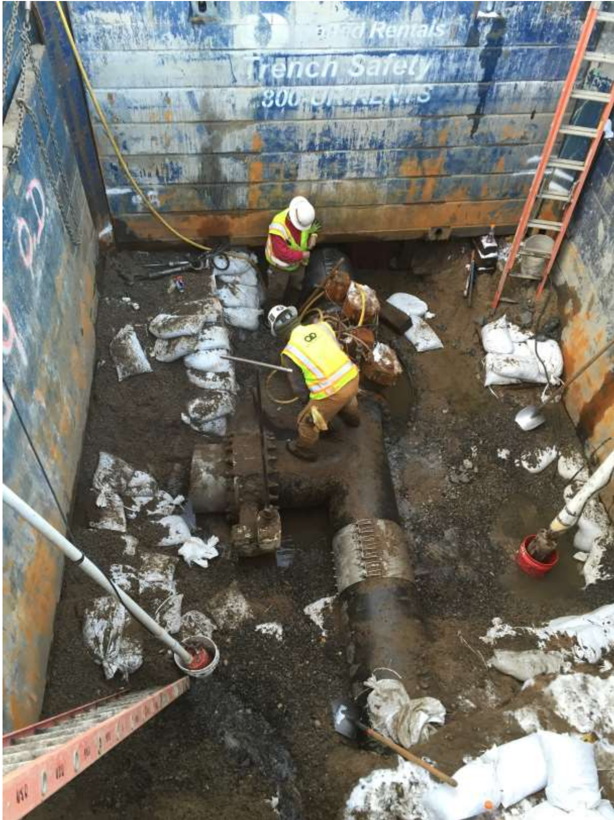
Existing T-section of HDPE pipe on intake line (photo courtesy of KGID)
