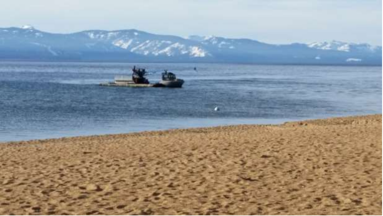
Dredging & weighting the intake line to get it back into place (photos courtesy of KGID)
