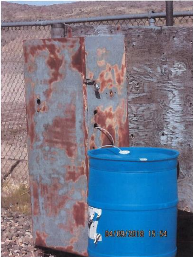
SCADA and Chlorination facility susceptible to vandalism (2018)
