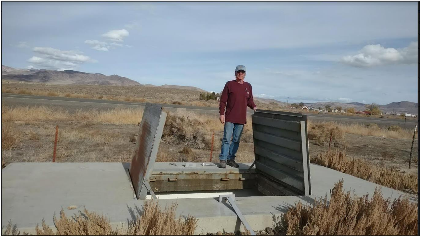
Staff showing the padlocked Vaults to distribution system adjacent to the highway
