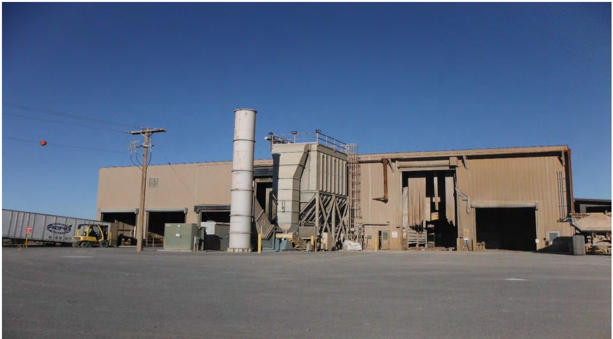
Photo 16-Treatment Pans 4 and 5, with dust control baghouse in the middle. An unloading dock to the Container Management Building is on the left.
