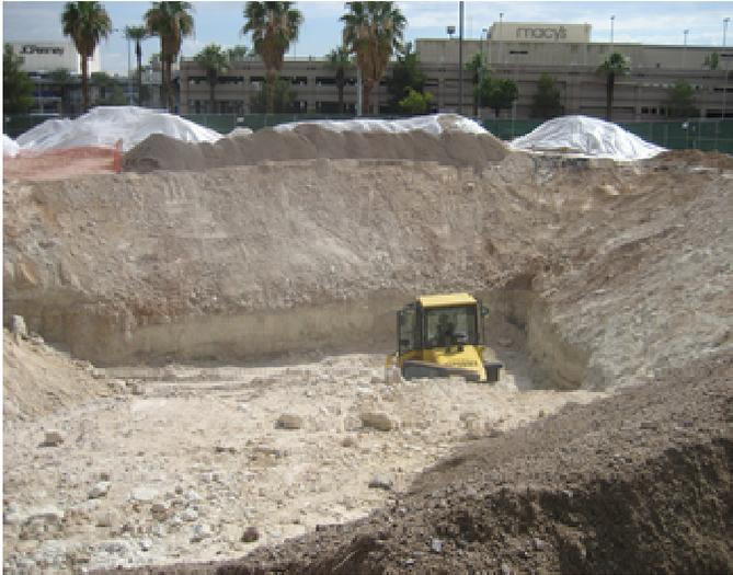
Application of oxidant on floor of excavation
