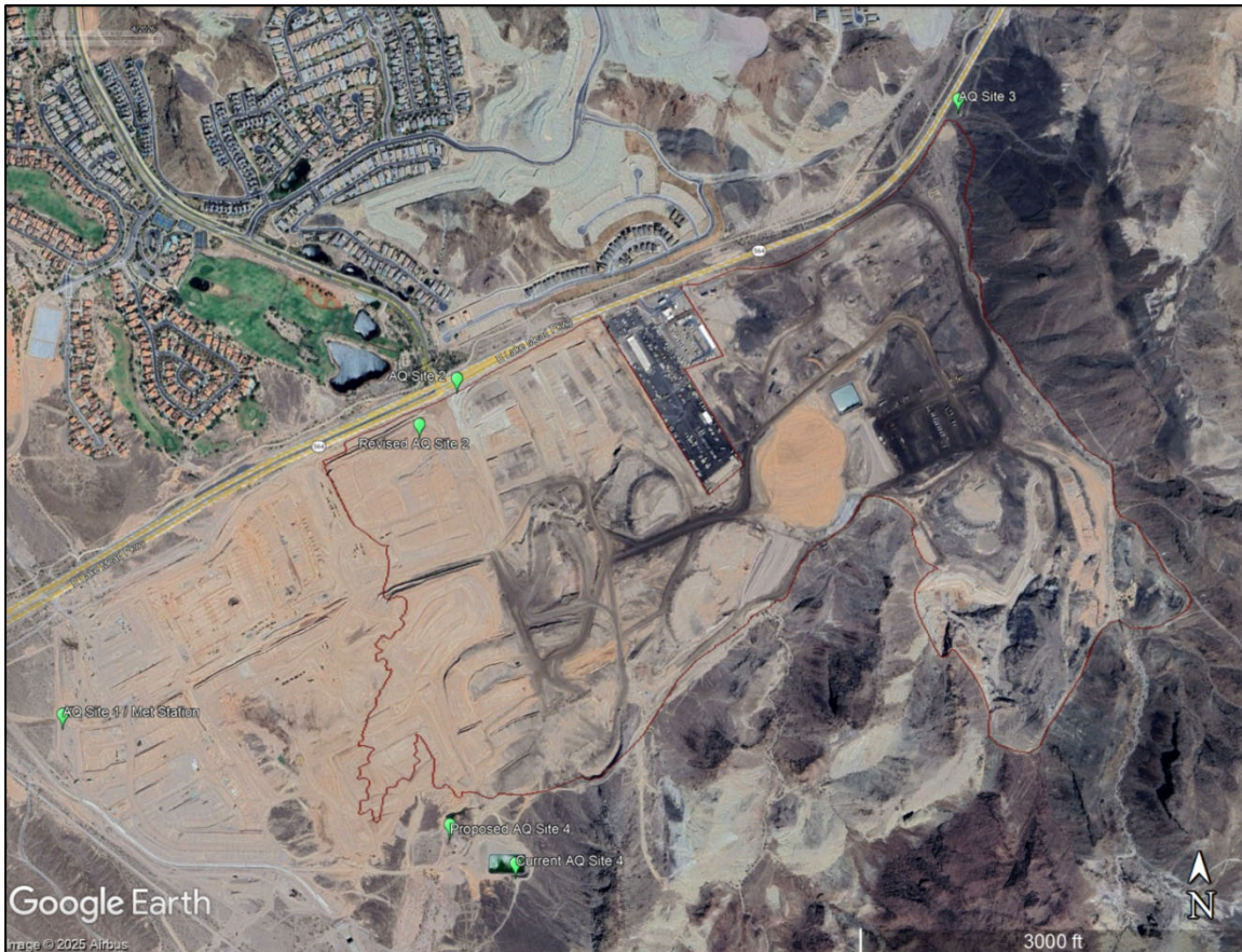
Figure 1 Monitoring Locations (Revised). Google Earth. Green pins depict perimeter air monitoring locations. The red line represents the impacted area of the former mine site.
