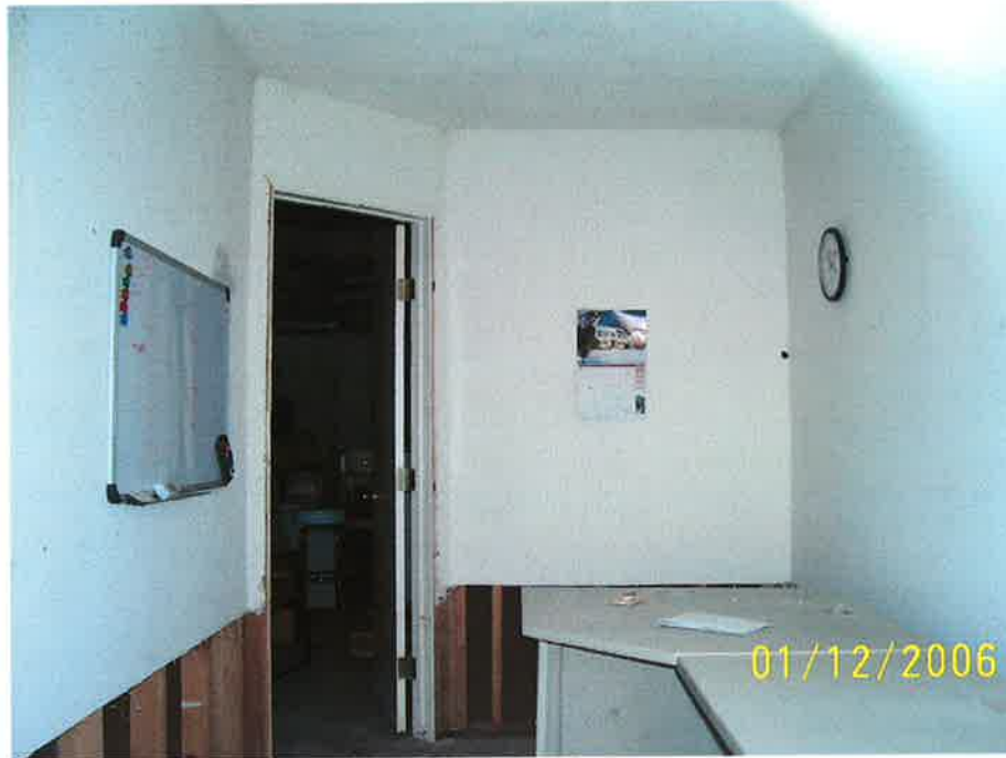
VIEW OF SMALL OFFICE IN SITE BUILDING. NOTE TRIMMED SHEET ROCK WALLS UNDER REPAIR FOLLOWING THE FLOOD OF 1-1-06.
