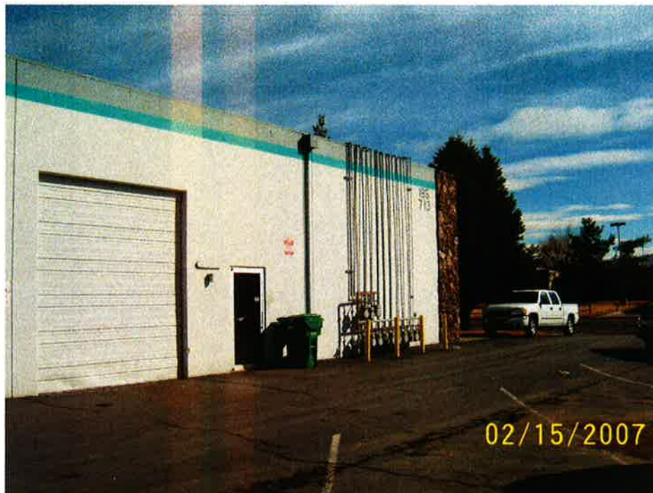
VIEW OF GAS METERS AT 185 N. EDISON WAY TYPICAL ON BOTH BUILDINGS.
