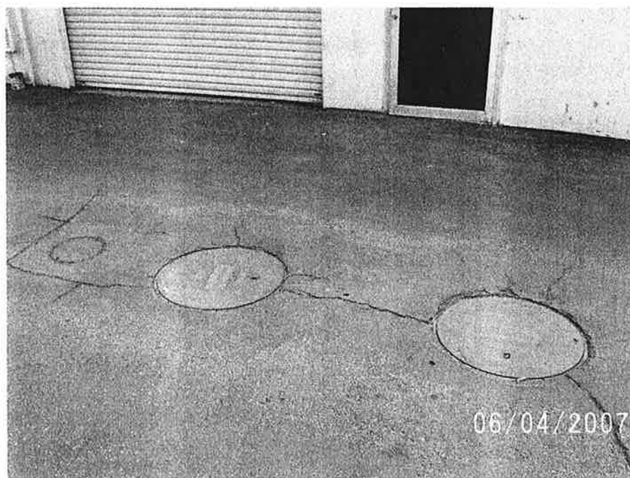
VIEW OF GREASE TRAP LOCATED ON THE EAST SIDE OF THE SITE BUILDING.
