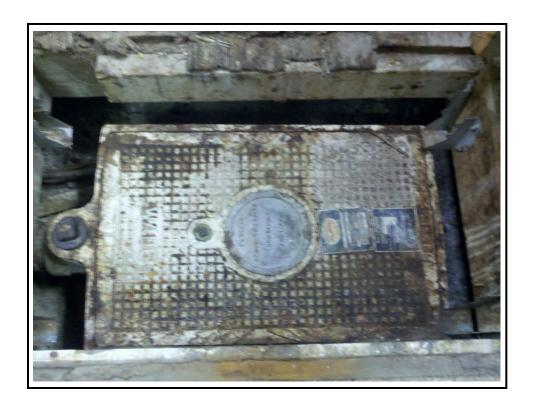
Photograph 17: Convention Center kitchen grease interceptor beneath floor
