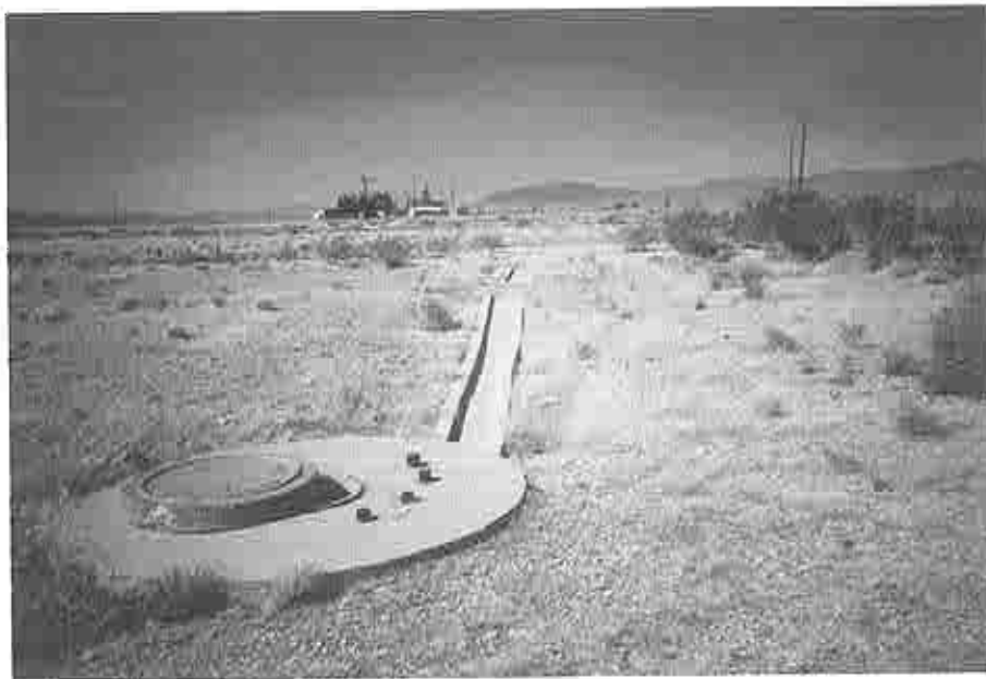
Photograph C-14: Oil/water sump located at the ACFS-Midway Street fuel island.
