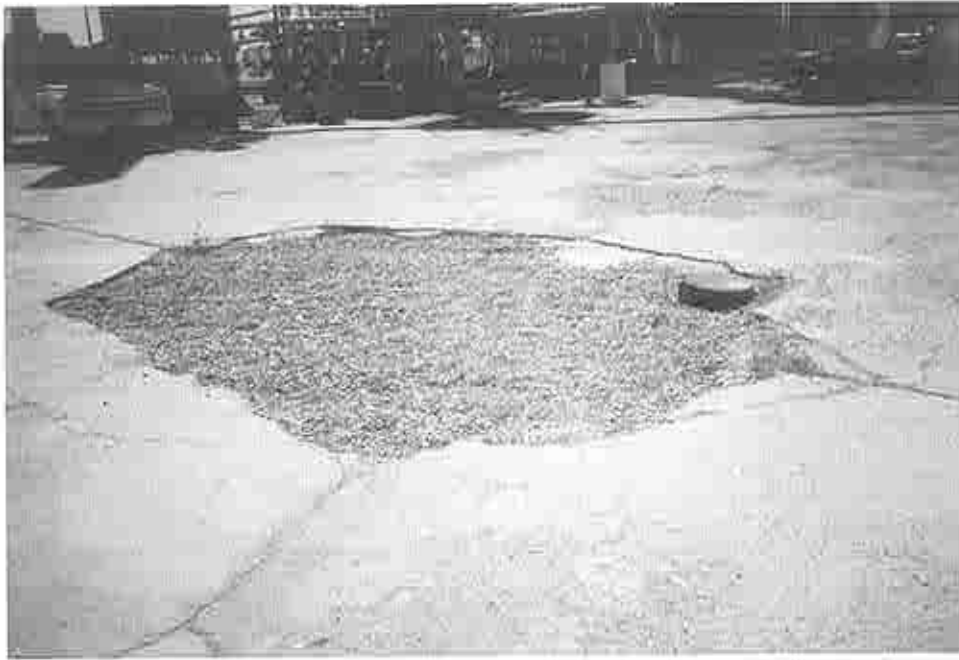
Photograph C-19: View of gravel-filled drain excavated through the former concrete slab of hangar Building 1600 used by the oil refinery for surface runoff drainage.
