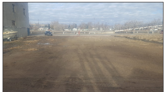
State Hotel property, post-demolition
