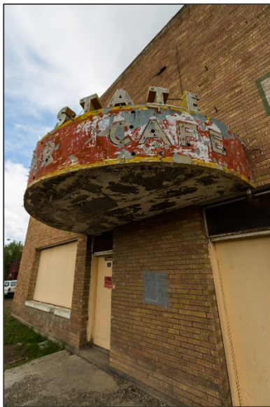
State Hotel, pre-demolition
