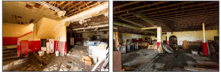
State Hotel, pre-demolition
