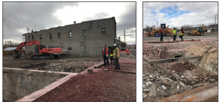
State Hotel, during demolition
