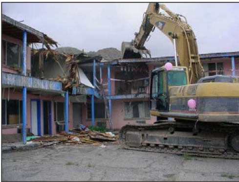
Building demolition following abatement
