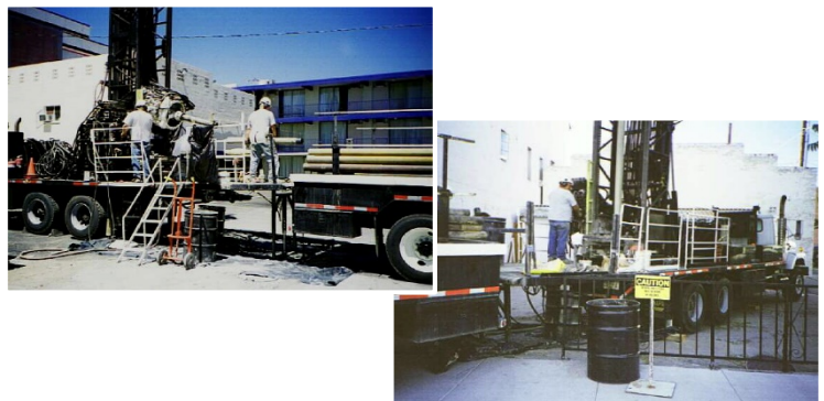
Technicians use a drill rig to install groundwater monitoring wells
