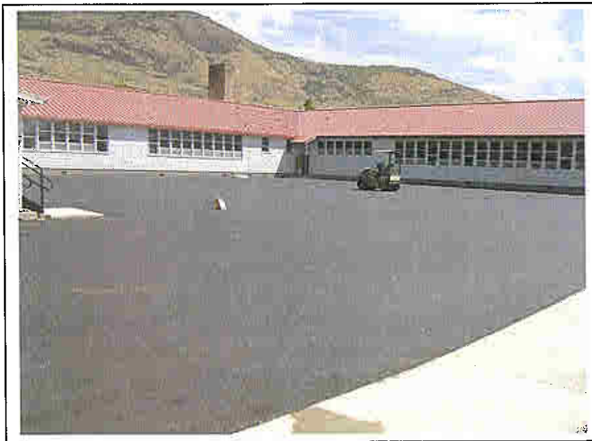
Photo 6: Final compaction of asphalt.
