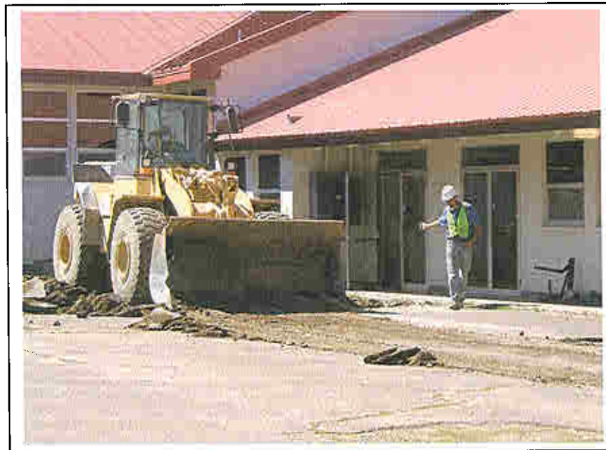
Photo 2: Asphalt removal.
