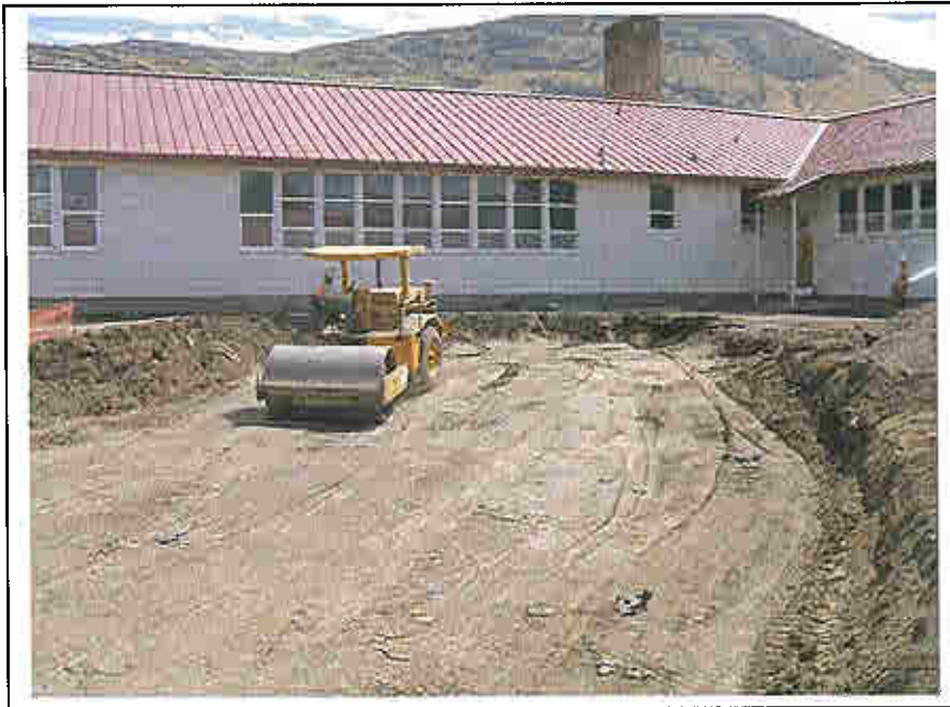
Photo 5: Excavation backfill compaction.
