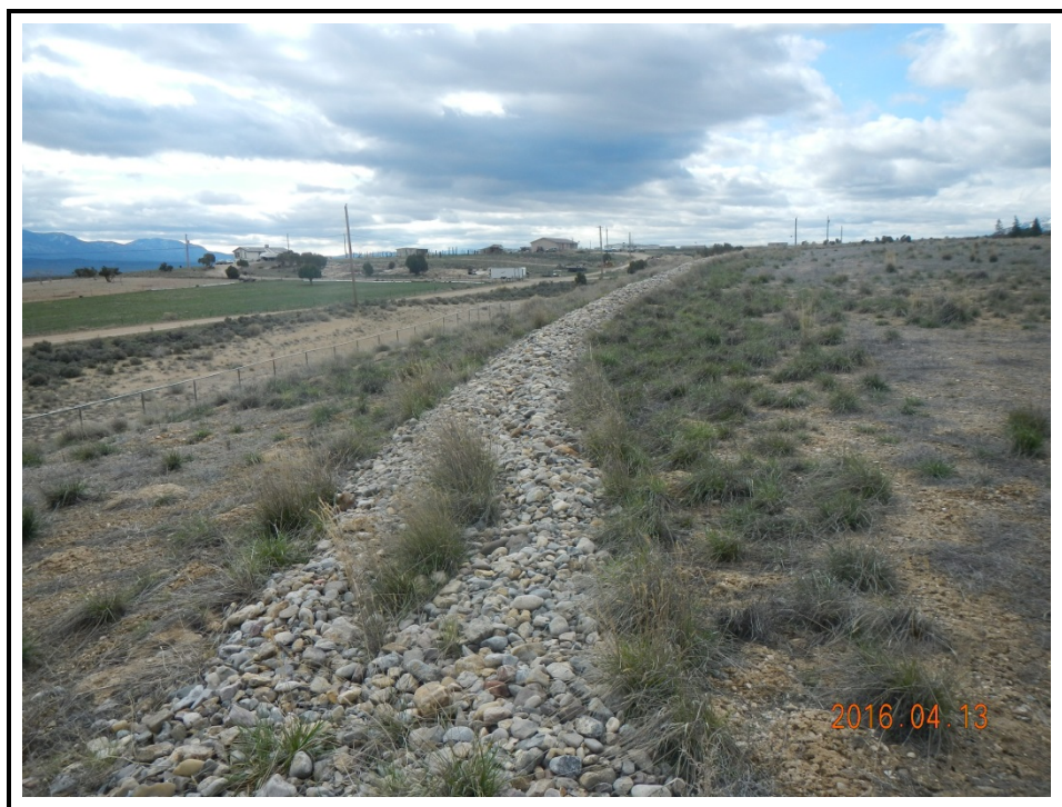
Photograph 13: View of rock berm on top of the covered landfill
