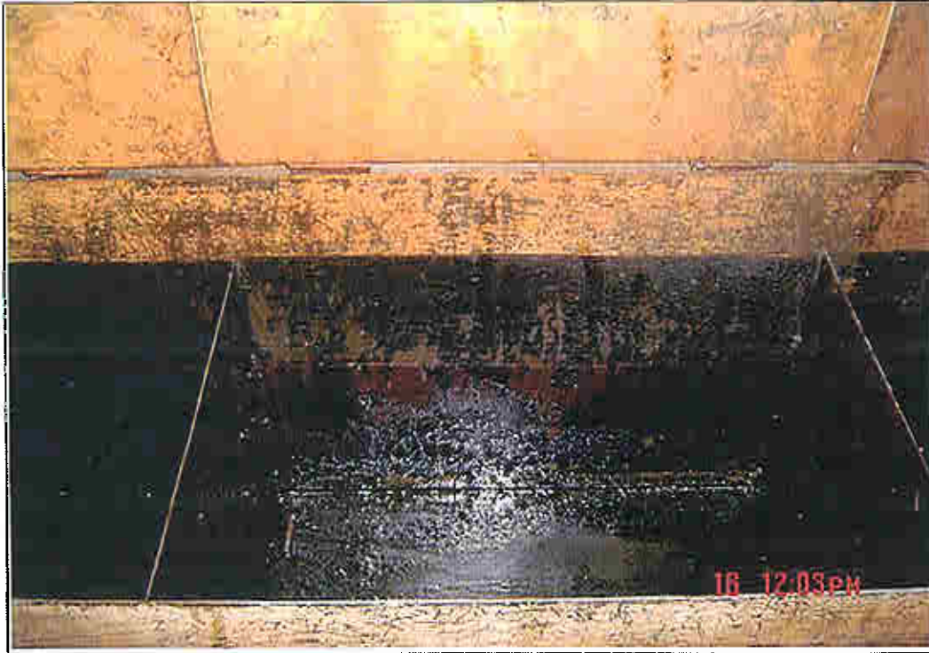
Photograph No.: 23 Photograph Location: Inside storeroom next to Engine Building Description: After Cleanup - Oil was also removed from the metal basin in the storeroom.
