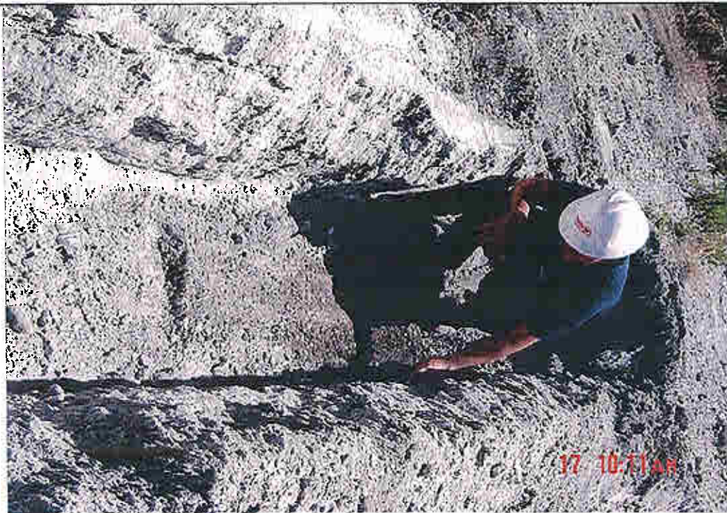
Photograph No.: 24 Photograph Location: Behind Engine Building Description: Lime layer of 2 feet deep was excavated and removed for disposal.
