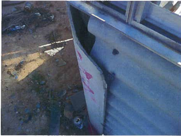
Suspect asbestos containing skirting along perimeter of greenhouse
