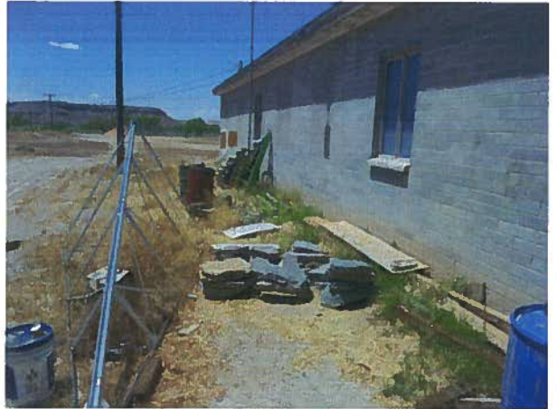
Looking south along east side of Senior Center building
