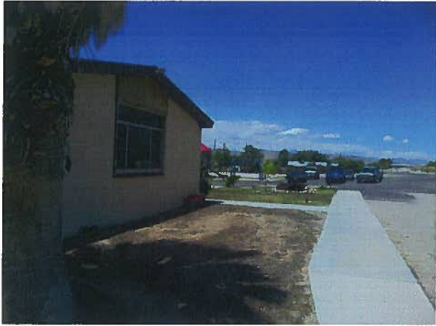
Looking west along north side of Senior Center building
