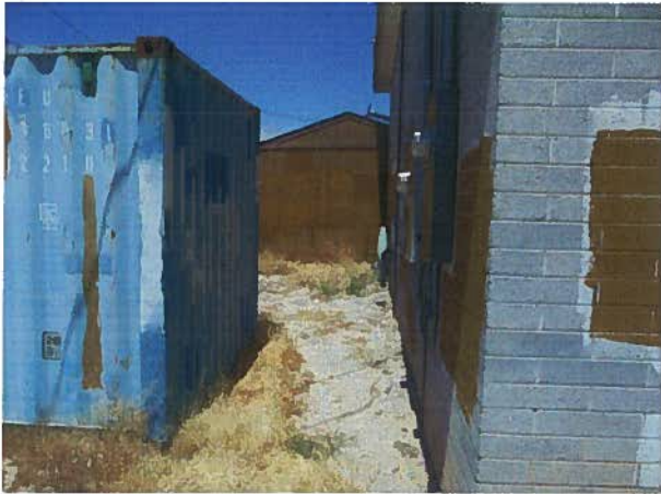
Looking west along south side of the Senior Center building
