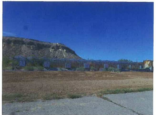
West adjacent Small Greenhouse
