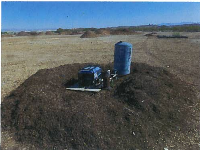
On-site groundwater well, with generator, west of Packing Plant
