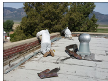
Asbestos abatement workers removing window putty (top photo) and roof mastic (bottom photo)
