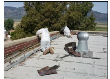
Asbestos abatement workers removing window putty (top photo) and roof mastic (bottom photo)
