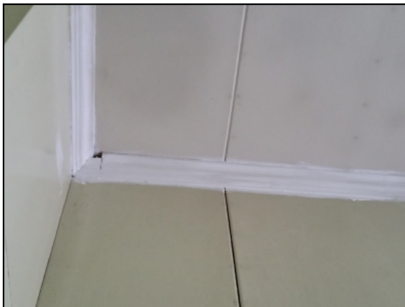
Picture 23—Crown molding in the men's room following prep ,including application of two stage lock down and primer.
