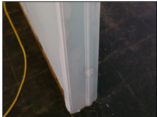
Picture 24—Door frame and casing between the kitchen and living room following prep ,including application of two stage lock down and primer.
