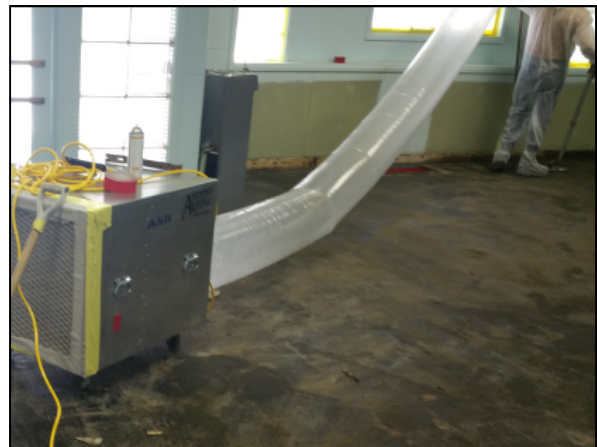
Picture 6—Interior of the containment, during VCT and base cove abatement. Negative air machine and worker using HEPA vacuum.
