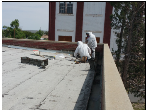
Picture 18—Workers removing the metal flashing that contains roof mastic and lead solder.
