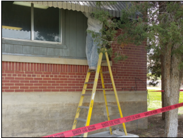
Picture 21—Worker scraping loose and flaking paint on the window trim on the west side of the building.
