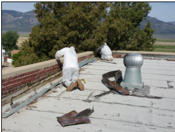
Picture 17—Workers removing the metal flashing that contains roof mastic and lead solder. Note: The black material remaining on the brick wall is non-asbestos containing tar.
