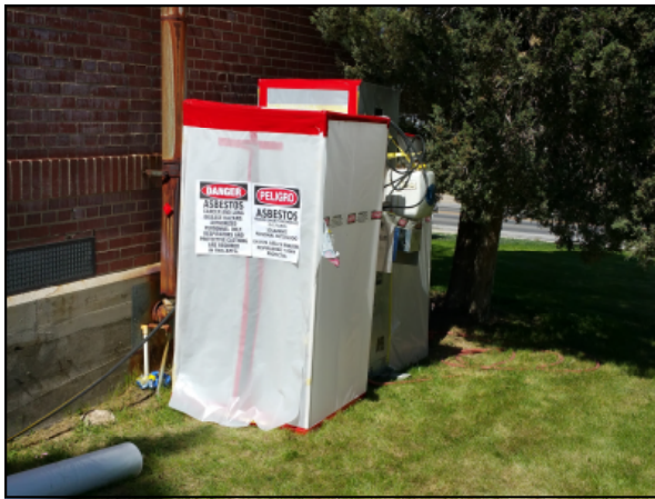
Picture 7—3-Stage decontamination chamber with shower, outside of the entrance to the basement.
