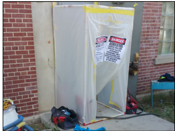
Picture 2—Outer, “clean room” stage of the decontamination chamber to the interior abatement.
