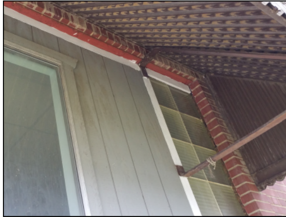
Picture 25—Window trim on the west side of the building following prep ,including application of two stage lock down and primer.
