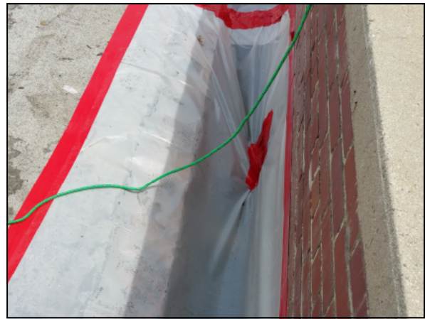
Picture 20—A&B constructed a temporary water barrier where the gutter had been, draining toward the downspout.
