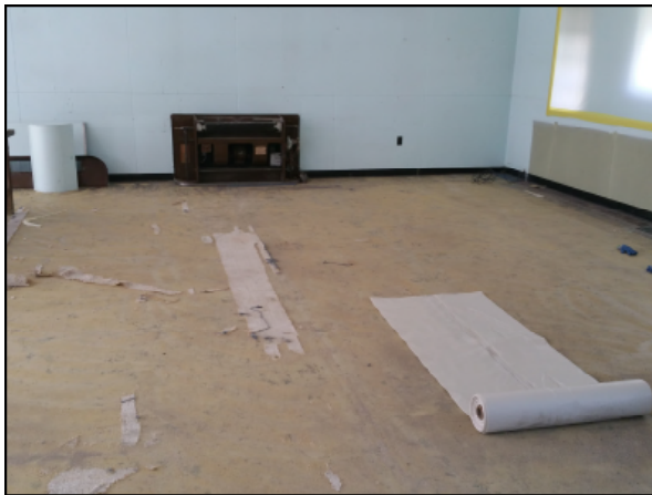
Picture 1—Interior of the building following carpet removal, prior to commencing VCT and base cove abatement.
