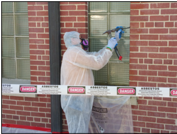
Picture 13—Worker removing window putty on the east side of the building.
