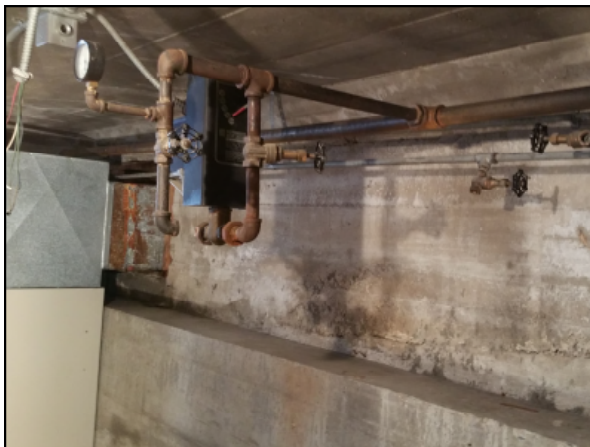
Picture 11—TSI removed and debris cleaned up in the basement.
