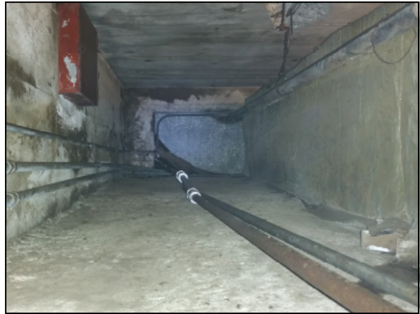
Picture 10—TSI and black mastic removed and cleaned in the north end of the North-Center crawl space.
