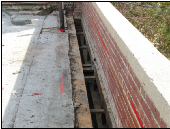
Picture 19—East side of the roof following the removal of the gutter. Note that there was no plywood or other barrier beneath the gutter.
