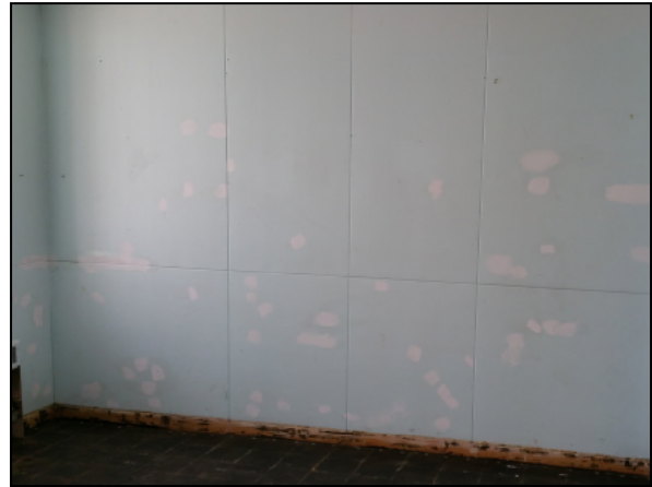
Picture 22—Wall inside the main room following prep of the fiber-board walls including application of two stage lock down and primer.
