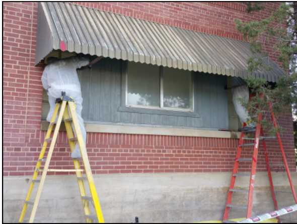
Picture 15—Workers removing window putty from the windows on the west side of the building.
