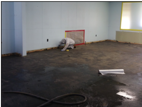
Picture 5—Worker conducting detail cleaning of the floor and lower walls in the interior of the building.
