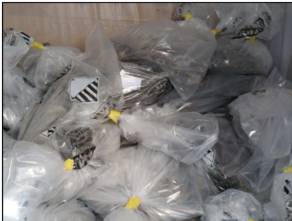
Picture 3—Bags of VCT and base cove debris.
