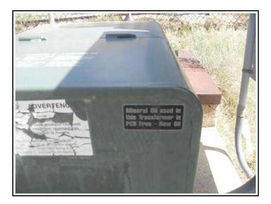
Photograph 25: Pad-mounted transformer PCB-free sticker
