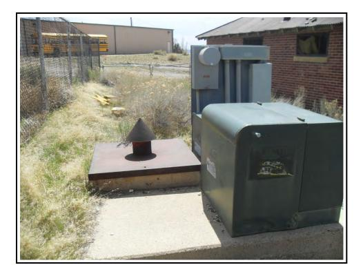
Photograph 24: View of paid-mounted transformers with utility vault venting system
