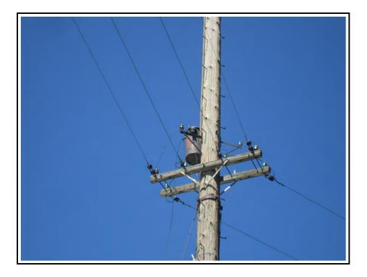
Photograph 27: Close-up view of pole-mounted transformer
