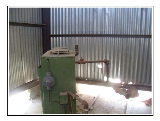
Photograph 31: Propane heater equipment in shed adjacent to bathroom (outside of fenced area)
