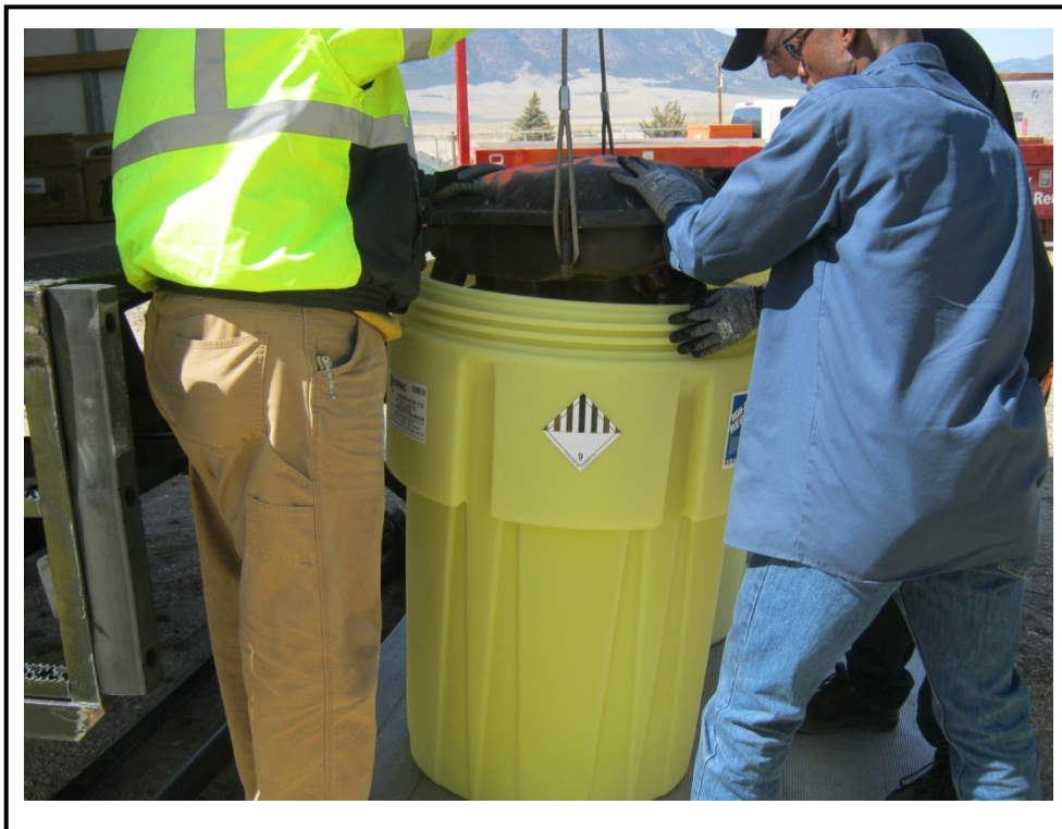
Secure intermediate storage of removed transformers
