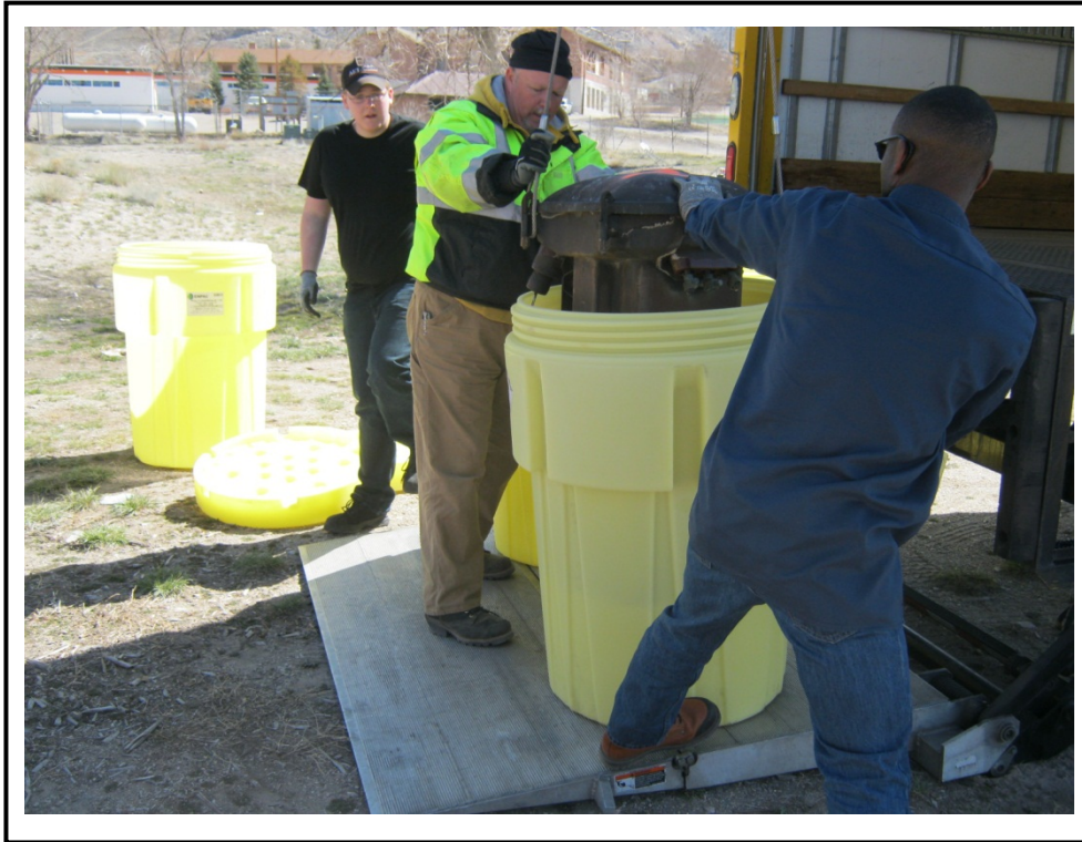
Placement of transformer into overpack drums
