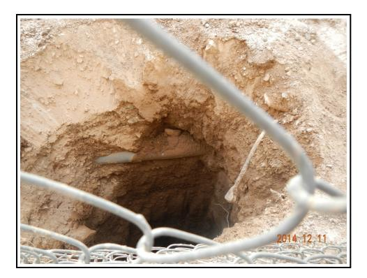
Observed excavation near northwest corner of Subject Property – appears to be associated with installation and/or removal of power poles
