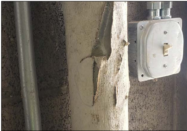
Identified damaged friable ACBMs (pipe insulation)
