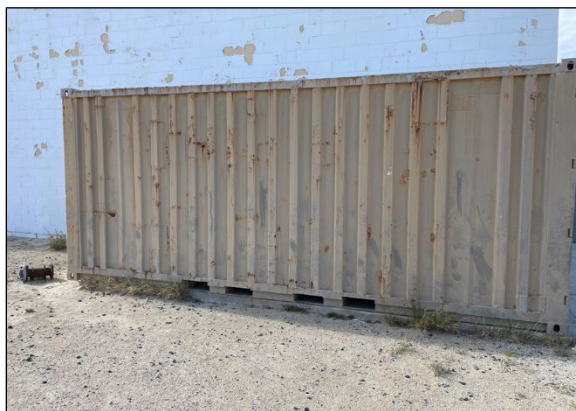
Metal storage container containing LBP on exterior surfaces
