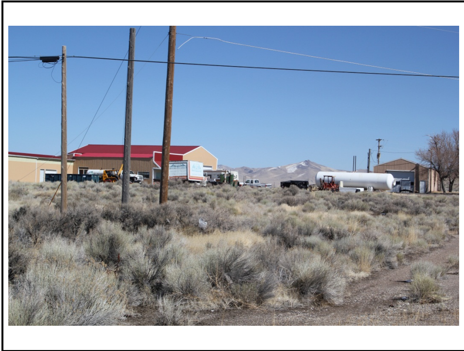
Photograph 7: Adjacent property to the east with several building structures
