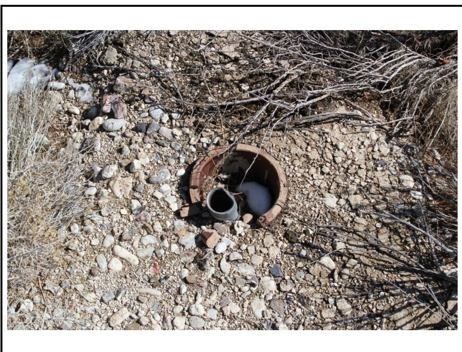
Photograph 14: Potential evidence of orphaned USTs (REC) on subject property—cover plate fixture containing buried conduit near unsurfaced road on subject property
