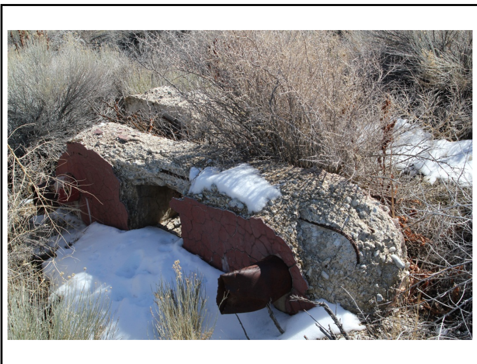
Photograph 13: Potential evidence of orphaned USTs (REC) on subject property--concrete section with metal bollard observed near unsurfaced road on subject property
