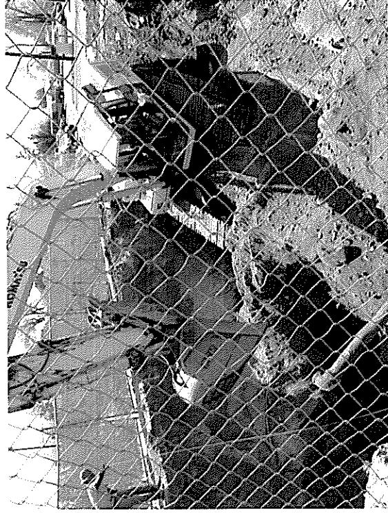
Photograph 6 – Collecting confirmation samples at 16 feet.
