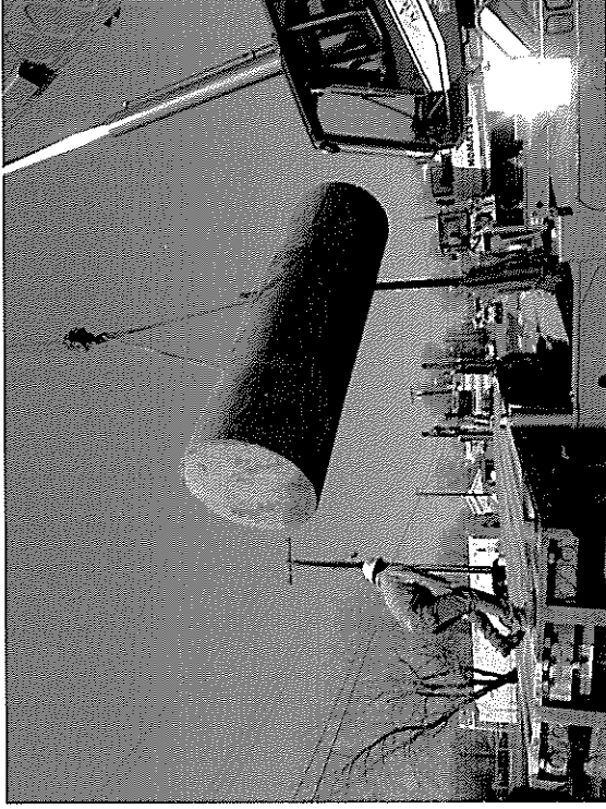
Photograph 3 – UST nearly to the trailer.
