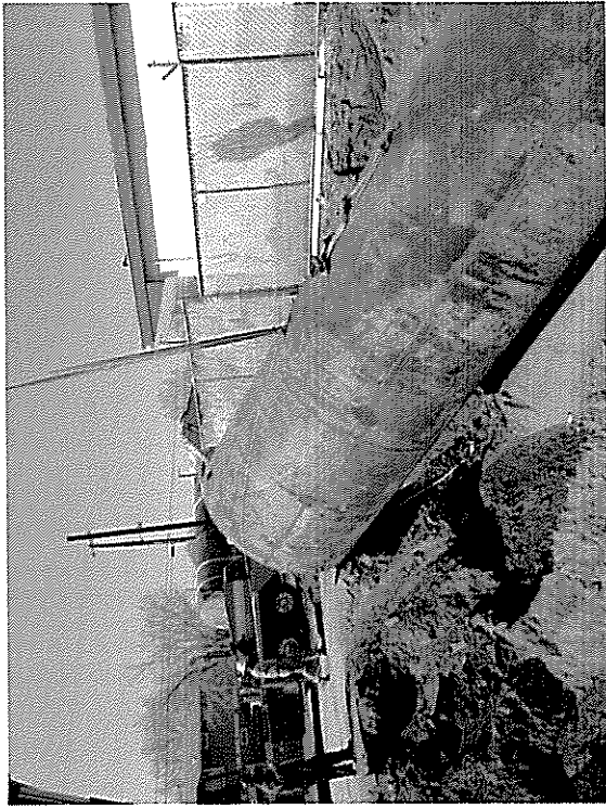
Photograph 1 – Preparing to lift one of the UST's.
