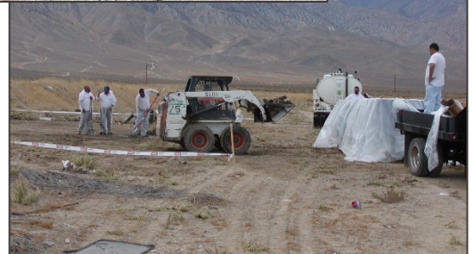
Asbestos containing materials cleanup
