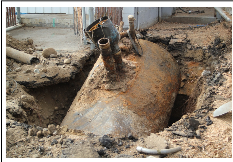
Waste oil tank ready for removal from excavation
