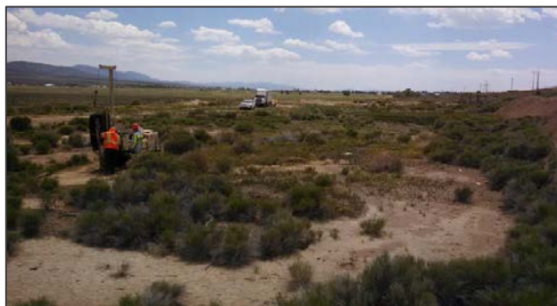
Workers take soil borings at the mill site
