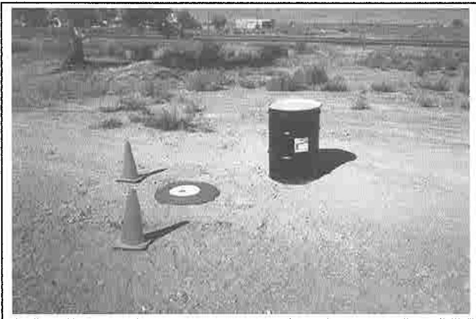
Photo 4: Completed monitoring well MW-1, near northwest corner Site. Drum contains investigation derived waste, soil cuttings.
