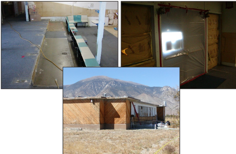
Above: Building during cleanup activities
