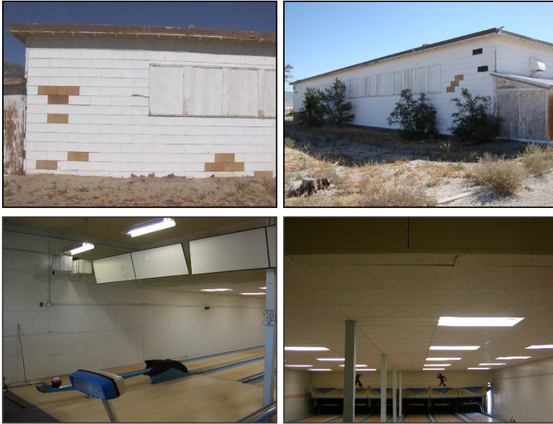
Above: Pre-cleanup building exterior and interior condition
