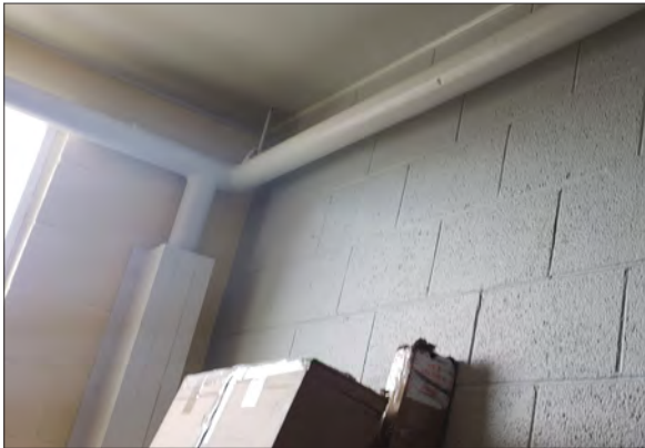
BGA25: White Fabric Coated Pipe Insulation.
