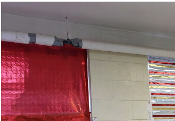
These pipes were considered "Occasionally" damaged according to AHERA terms for damage severity.
