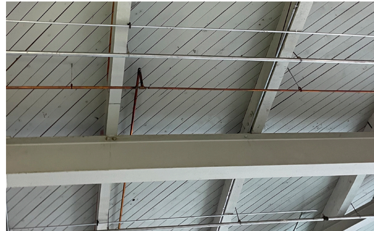
Lead chip sample Pb-06 was taken from green ceiling beam with intact paint.
