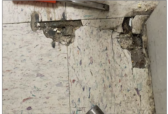
ACM was found in black mastic sample layer of HA BGA1.
