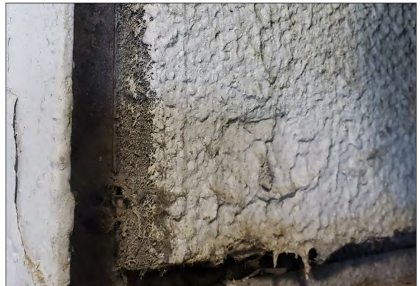
ACM was found in the black tar with paint layer of sample HA BGA7.
