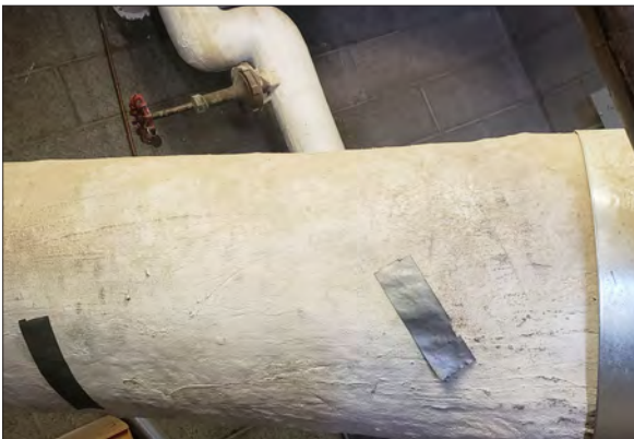
BGA16: White Fabric Pipe Insulation consisted of the pipe insulation that surrounded the boiler, and the pipe near the entrance of the Boiler Room.
