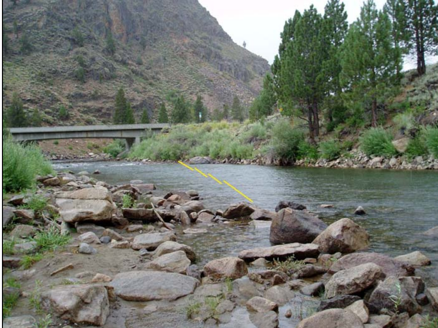
Site: West Walker River Site # WW1 – Sonora Bridge (Photo from taken south bank, looking upstream at bridge)
