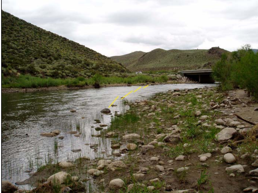
Site: West Walker River Site # WW2 – West Walker Bridge (B47-11) (Photo taken from west bank, looking upstream)
