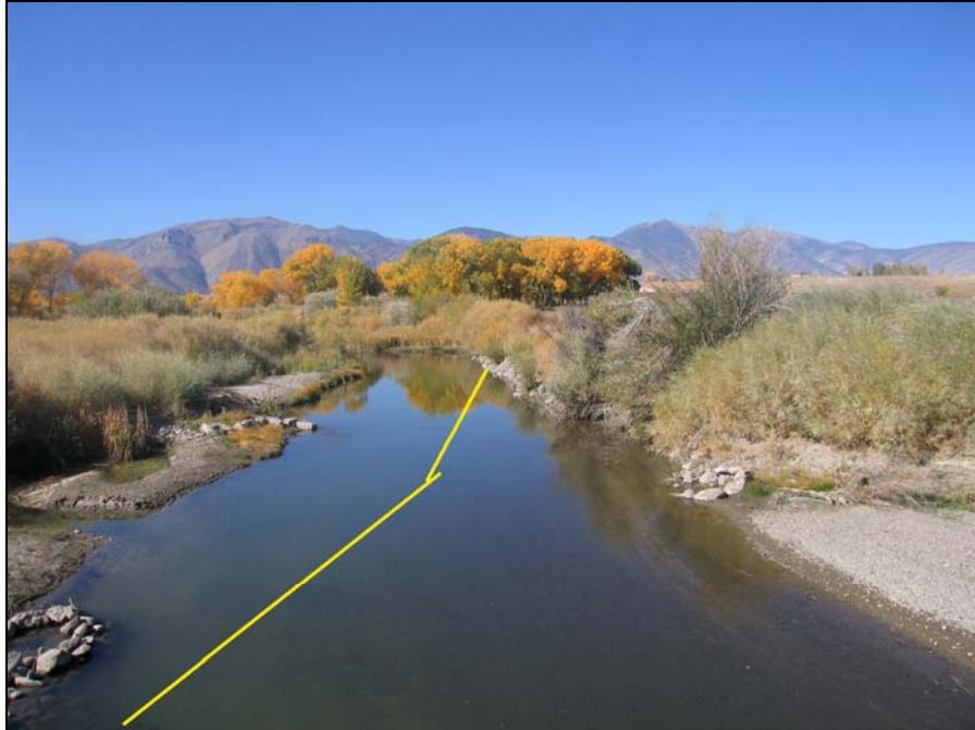
Site: West Walker River Site # WW15 – Smith Valley Bridge (B-822) (Photo taken from bridge, looking upstream)
