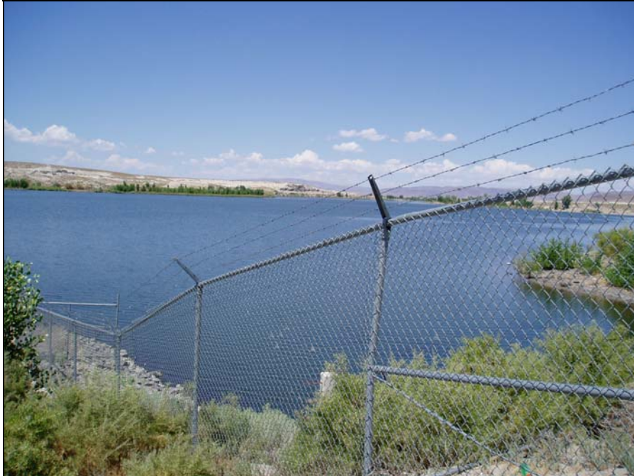
Site: Walker River Site # WR10 – Weber Reservoir Dam (Photo taken from bridge, looking downstream)
