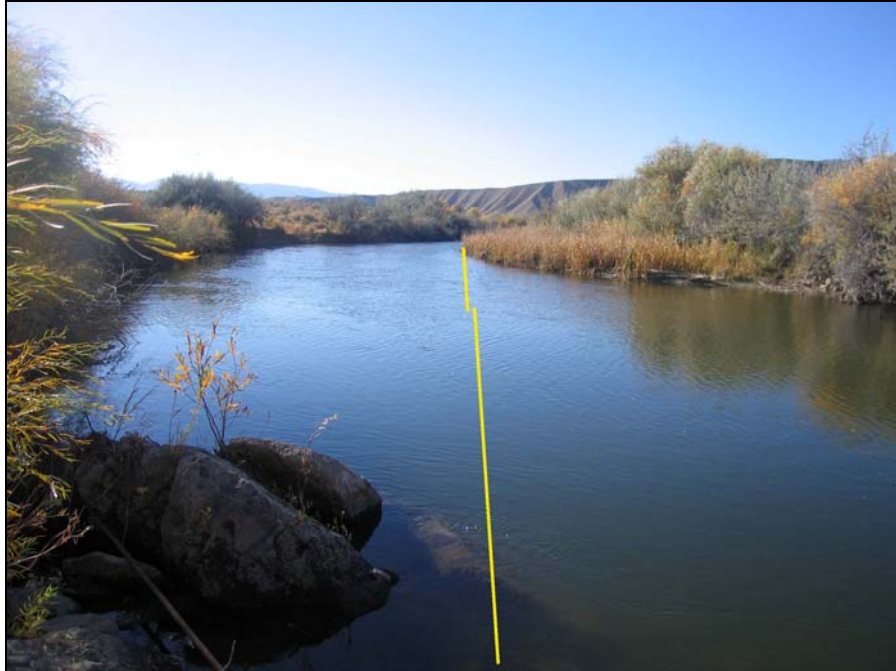
Site: West Walker River Site # WW13 – Hoye Canyon Diversion #1 (Photo taken from diversion dam, looking upstream)
