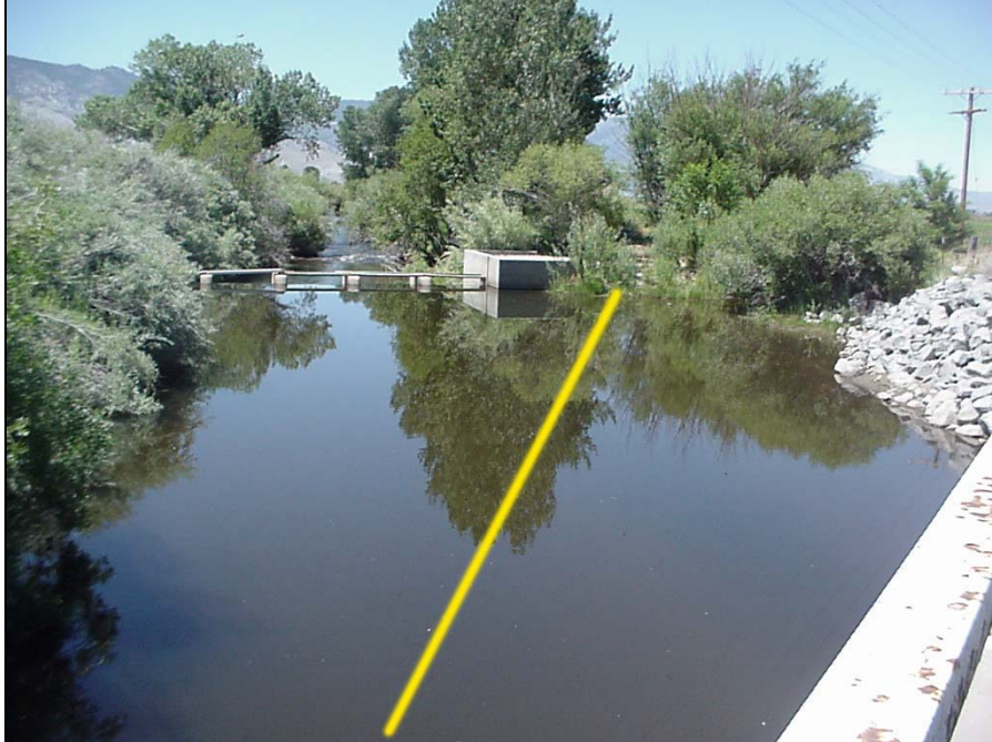
Site: Brockliss Slough Site #BR2 - Highway 88 Bridge South (photo taken from bridge, looking downstream)
