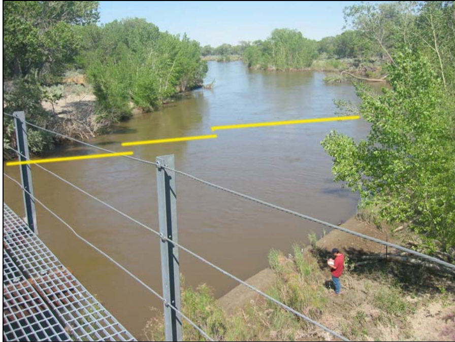
Site: Carson River Site #CR18 – Union Pacific Bridge (photo taken looking downstream from trestle)
