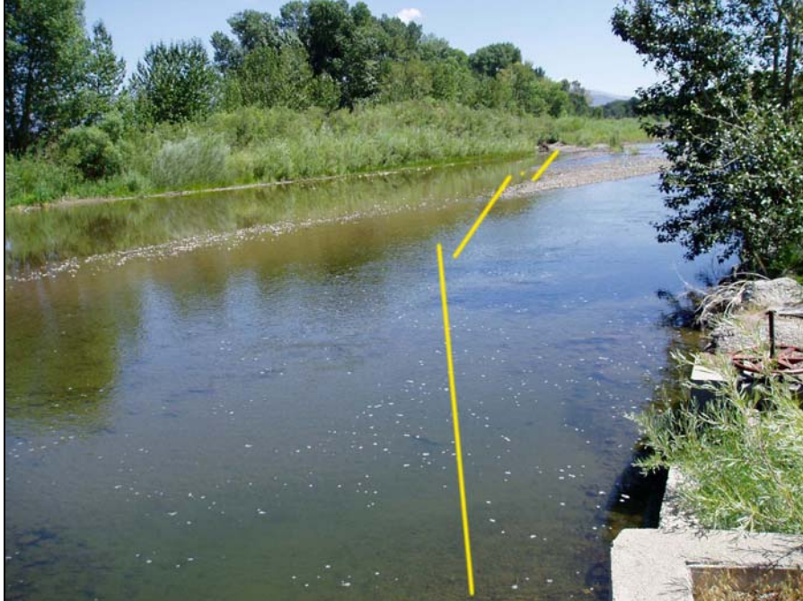
Site: East Fork Carson River Site #EF5- Cottonwood Ditch/Henningsen Ditch (photo taken from west bank, looking upstream)
