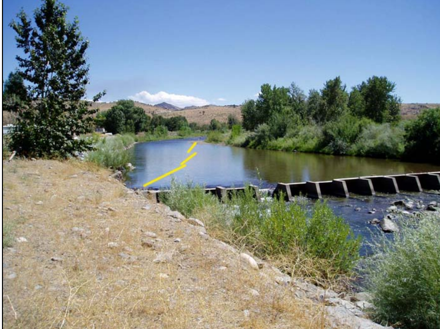
Site: East Fork Carson River Site #EF3- Allerman Canal (photo taken facing upstream, ditch gate is left of dam)
