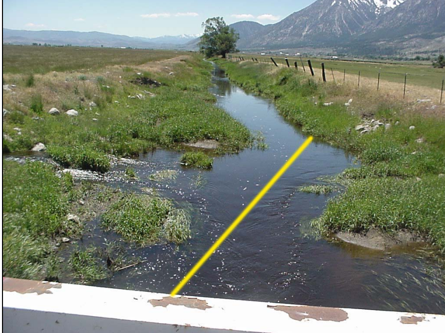
Site: Brockliss Slough Site #BR5 – Muller Lane Bridge 474 (photo taken from bridge, looking upstream)
