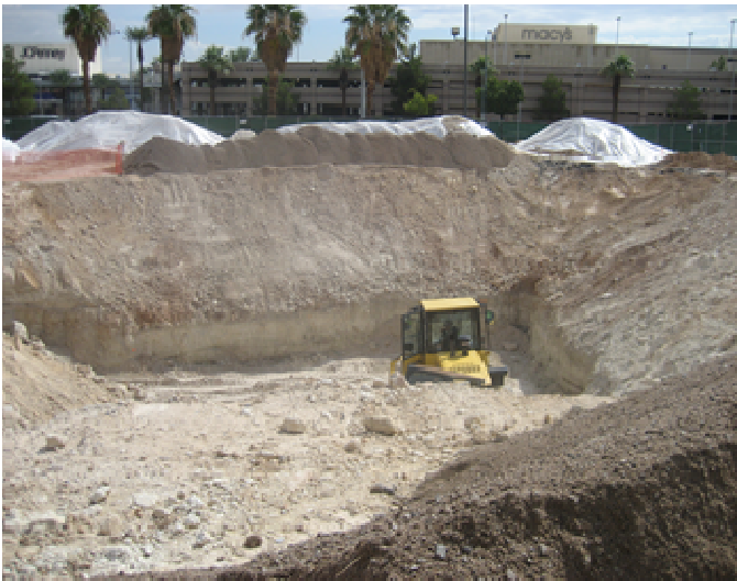
Excavation of source area soil - September, 2011
