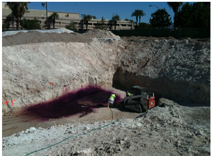
Application of oxidant on floor of excavation.
