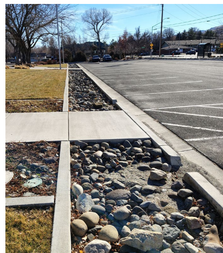
Curb cut and retention practice in parking lot. (Carson City, NV; Source: Carson City Public Works)
