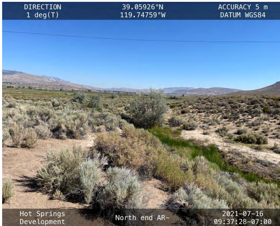
Photo 3. View of AR-1 at northern property boundary. Installation of concrete open bottomed box culvert will impact approximately 19 LF of stream will be reconstructed and realigned beneath the culvert. Culvert footings will permanently impact 902 SF of AR-1b of emergent wetland.
