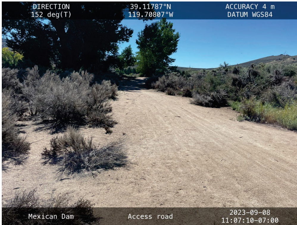
Photo 7: Existing access road. Adjacent dead vegetation (shown on left) to be cleared and area widened for equipment staging during construction.
