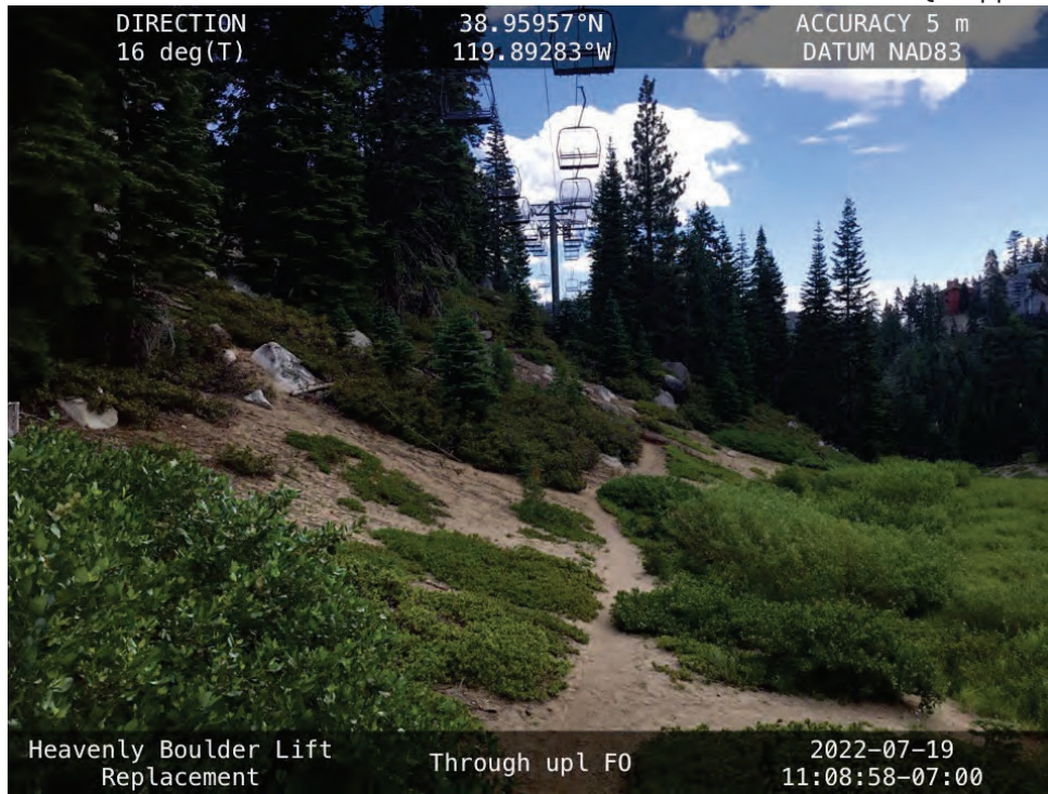
Photo 5. Construction access will utilize existing routes and disturbance corridors through upland forest when available.
