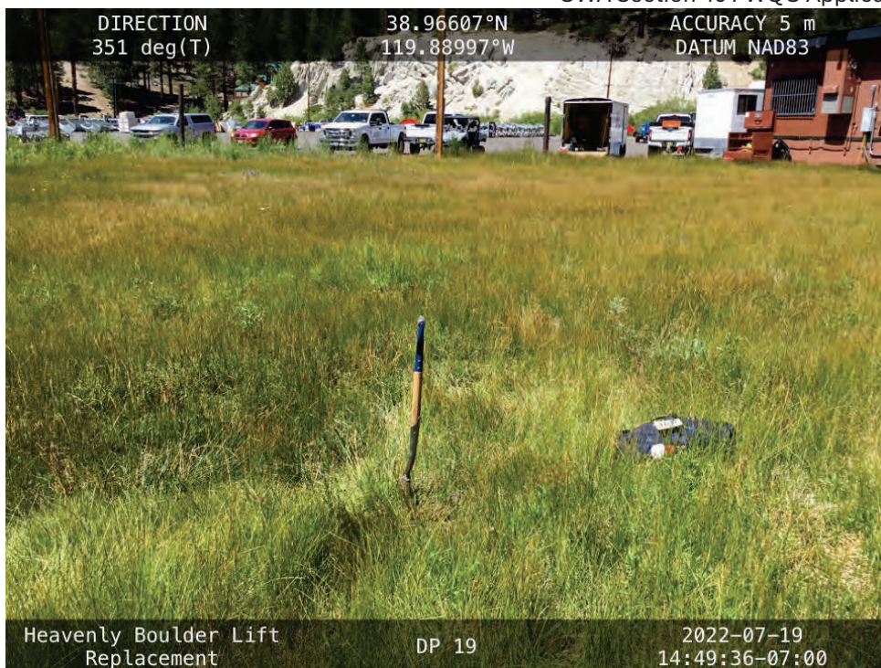
Photo 9. Project proposes to replace approximately 130 linear feet of an existing power line from the boulder lot through existing emergent wetland to the new lower lift terminal. Upon completion, the utility line trench will be back filled, wetland sod replaced, and temporary impacts to wetland will be restored to preconstruction elevation. No permanent impacts from replacement of existing power line.
